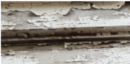
"Alligatoring" paint does not necessarily indicate that the surface below is damaged.
