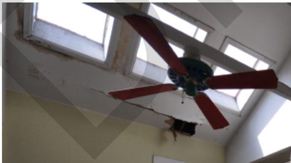
Skylights can cause extensive water damage if improperly installed and sealed, and are generally not recommended unless necessary to increase living space.
