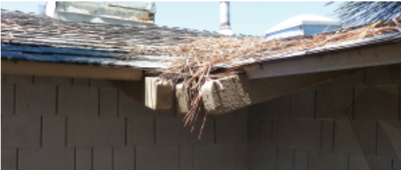
Excessive debris should not be allowed to accumulate.
