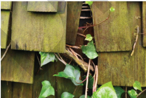
Algae and mold should be scrubbed away with a soft brush and gentle cleaning solution.
