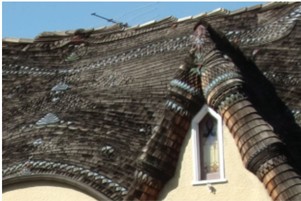
Significant and distinctive wood shingle roofs, like this wave-coursed roof with rolled eaves, should be preserved.
