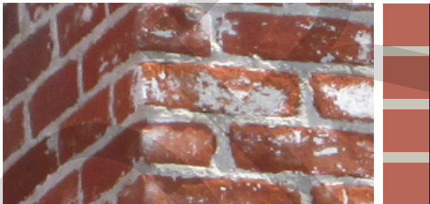
Flush Mortar Joints
