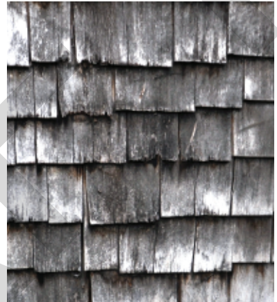
Without regular applications of wood stain, wood elements like these shingles are susceptible to warping, cracking, moisture, and even insects.
