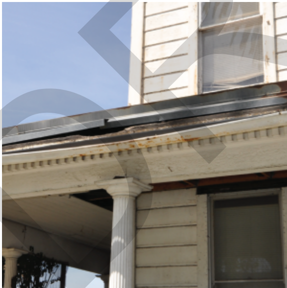
Broken, crooked, or damaged downspouts and gutters will not properly divert water away from a building.
