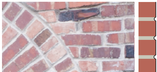
Recessed Mortar Joints
