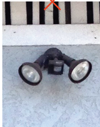
Contemporary lighting, such as the flood light pictured on the right, should not be used on the front elevation of a historic home.
