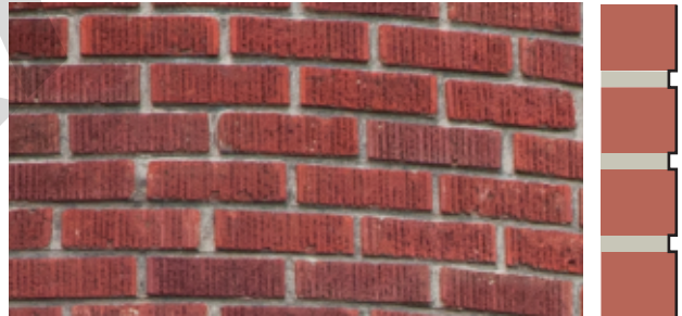
Raked Mortar Joints
