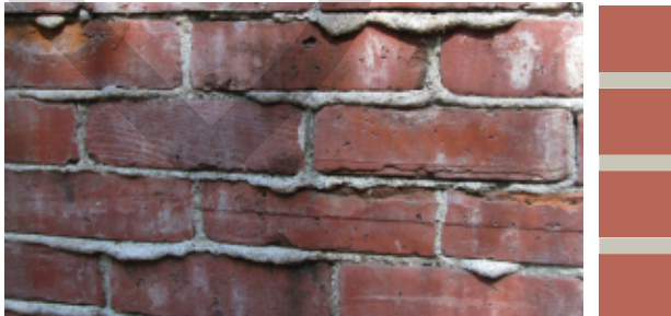
Oozing/Weeping Mortar Joints
