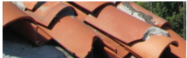
Clay tiles are susceptible to cracking, chipping, and breaking if handled without care.
