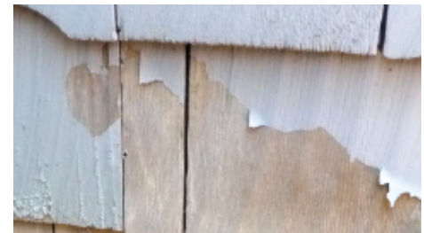
Paint is unlikely to adhere to an improperly prepared surface.
