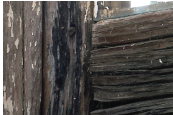
Wood rot, caused by moisture and certain types of fungus, may be damp to the touch and cause the wood to splinter away or break off in "chunks." It is typically easy to penetrate with an implement such as a pencil.
