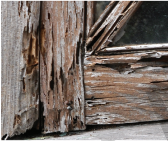
Left unchecked, wood-boring insects can cause irreparable damage to wood elements over time.
