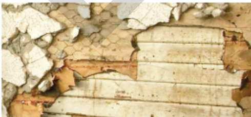
This wood siding was inappropriately covered in a layer of stucco.
