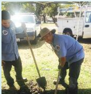
Facility Maintenance staff members Sabino Rodriguez, Marvin Cruz and Jorge Marentez fixed a broken water line at Cherry Park. They shut off water, cut out the broken pipe section, installed coupling, and had the site up and running within two hours of the call.
