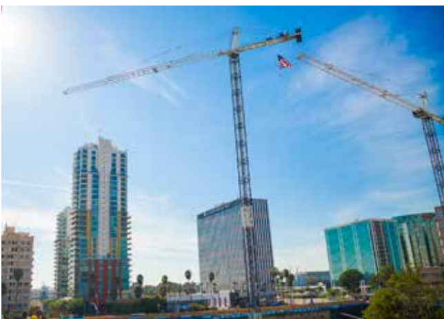
Construction of city hall
