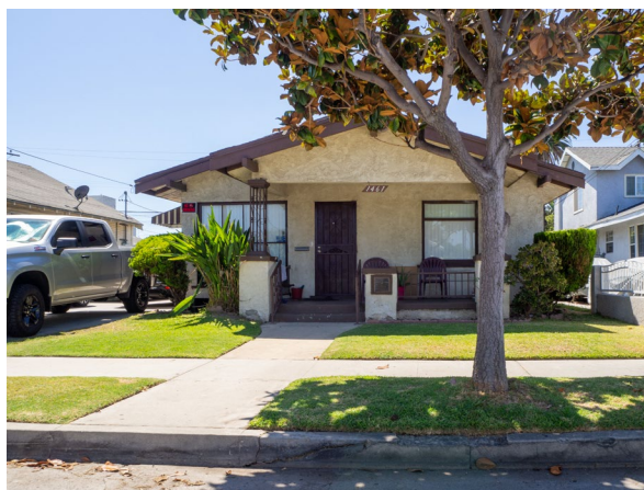
Figure 10. Ernest S. McBride residence, 1461 Lemon Avenue, 2020. Source: Historic Resources Group.
