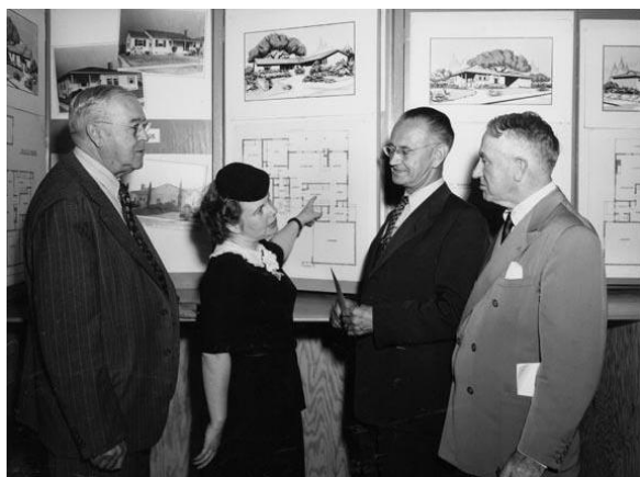
Figure 14. Lloyd Whaley (right) and others gathered around plans for Los Altos Manor, no date. Source: Historic Long Beach .
