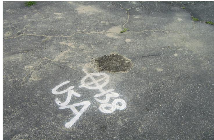
Photograph 16: View of the USA markout and an asphalt patch from soil boring B8 located in the parking lot adjacent to the south of the 5875 Atlantic Ave. site building.
