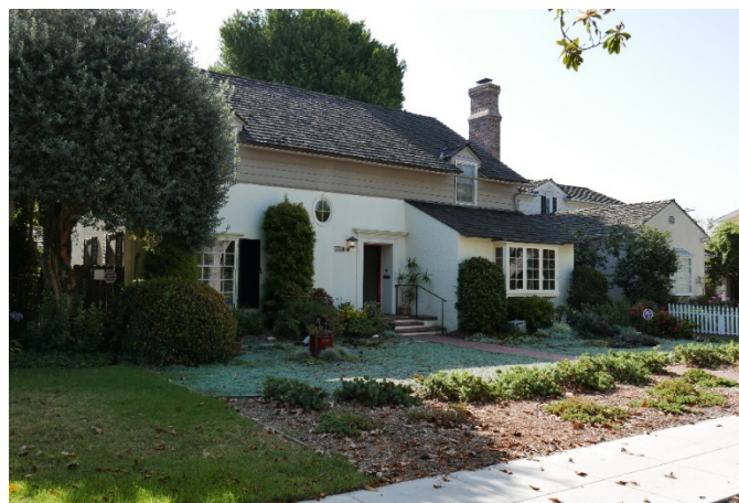
Primary (Western) Façade, 830 Santiago Avenue
