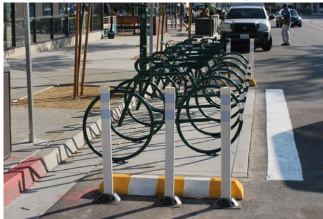
Bike parking is extended out into street parking stall.
