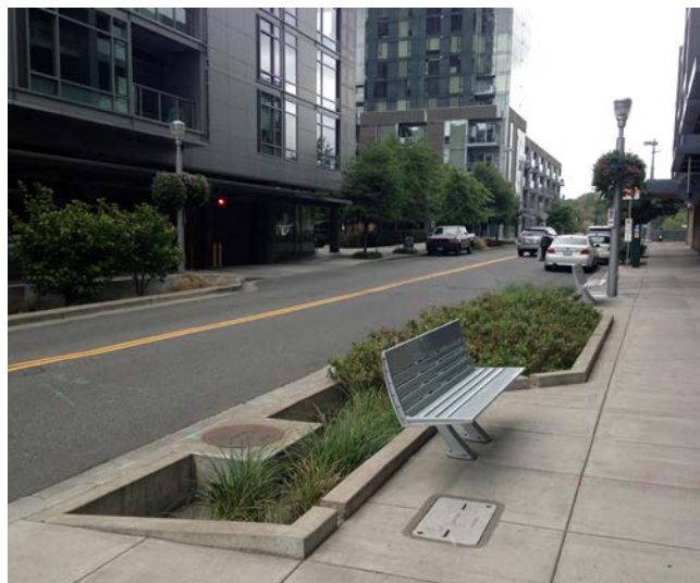
A bioswale filters stormwater before entering storm drains.
