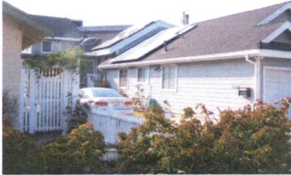
HPO pushed back the solar system from the best, sunny location in the front of the Ward home, to the rear, broken into three less-productive arrays.
