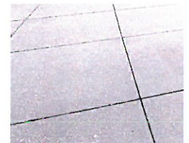
17 CONCRETE WALKWAY FINISH: MEDIUM BROOM FINISH COLOR: NATURAL GRAY BY: GENERAL CONTRACTOR
