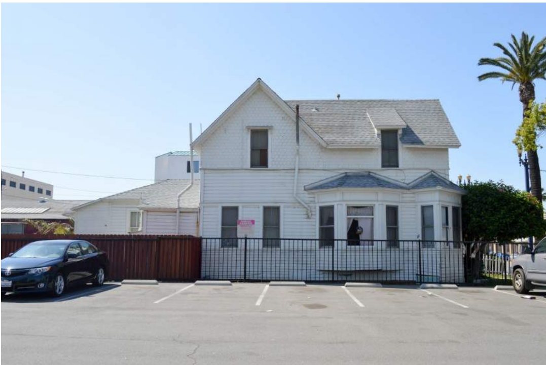
Parsonage Residence, North Elevation, View South, Photo: 2017.
