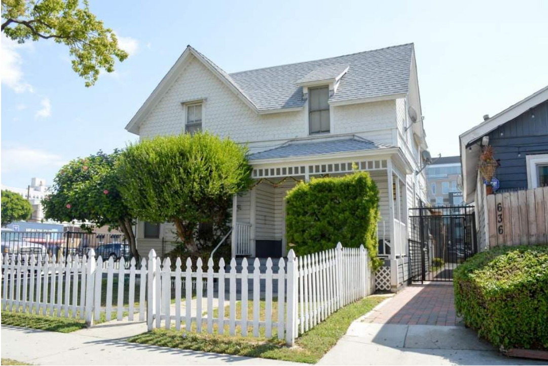
Parsonage Residence, Primary Elevation, View Northeast, Photo: 2017.
