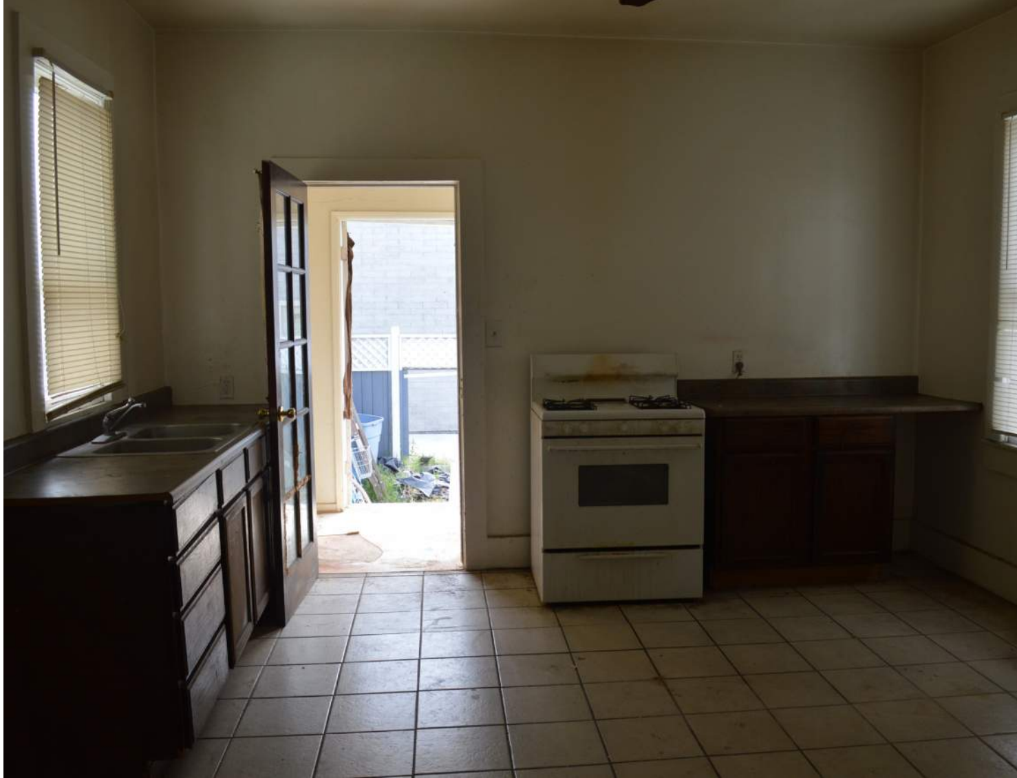
Kitchen area, First Floor, View East (existing condition) Photo: June 2018
