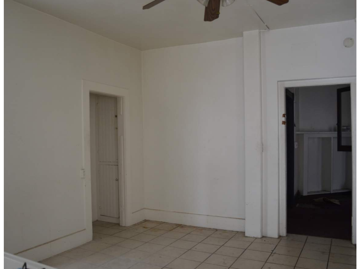
Kitchen, First Floor, View Southwest (existing condition) Photo: June 2018
