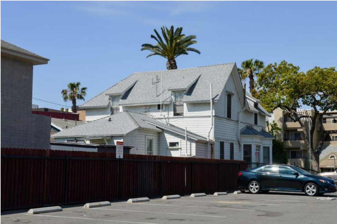
Parsonage Residence, East Elevation, View Southwest, Photo: 2017.
