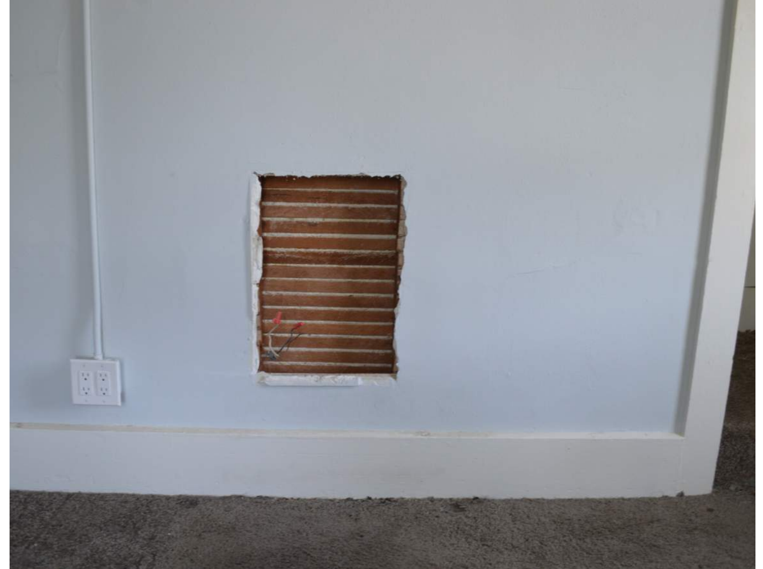
Original construction detail, Second Floor (existing condition) Photo: June 2018
