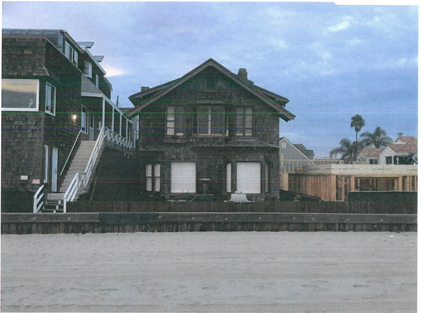
Front (South) view of 5719 E. Seaside Walk
