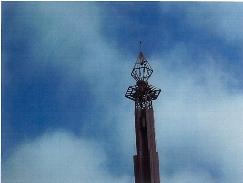
Subject Property – Cell Tower (Flat Panel Antenna)
