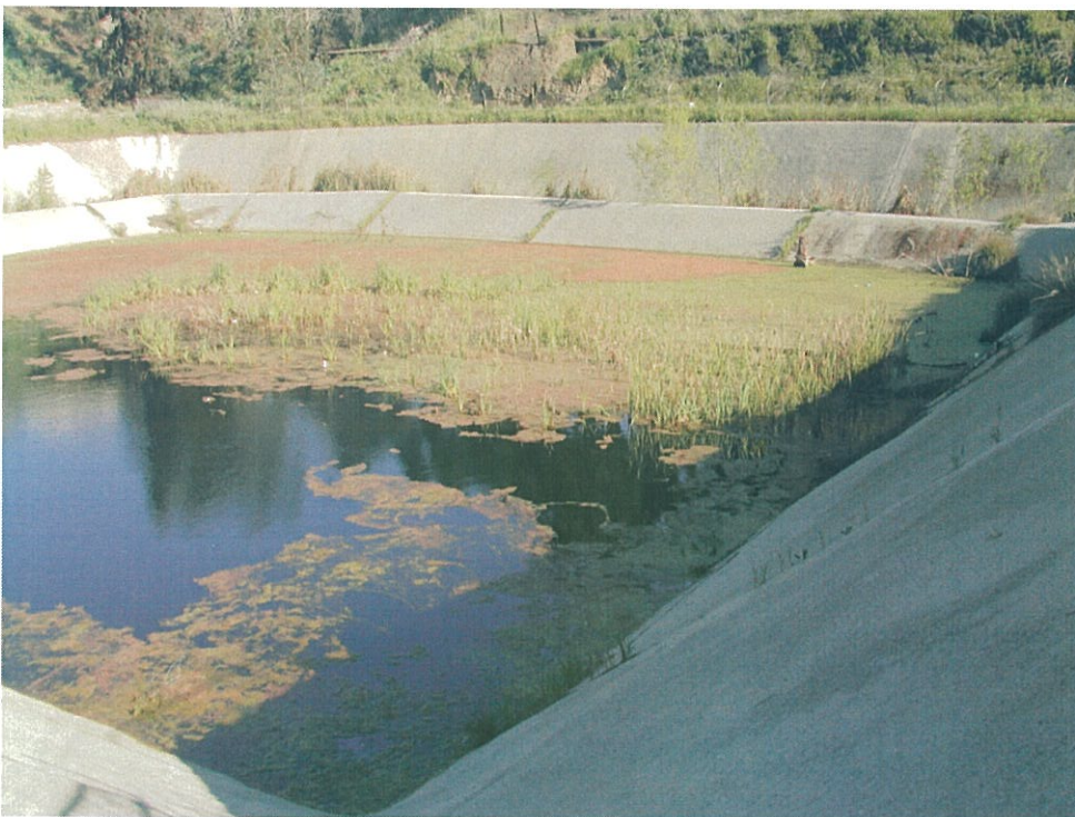
View to the southeast across existing retention basin.
