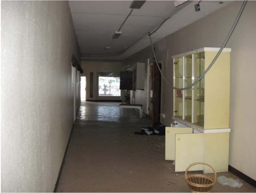
15. Interior finishes at the former church main hallway.
