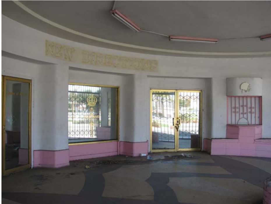
9. Exterior lobby of theater building.
