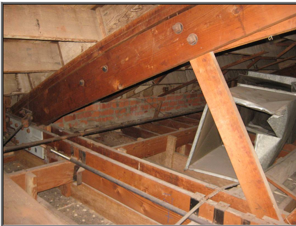
Photo 5: Typical strengthened bowstring truss.
