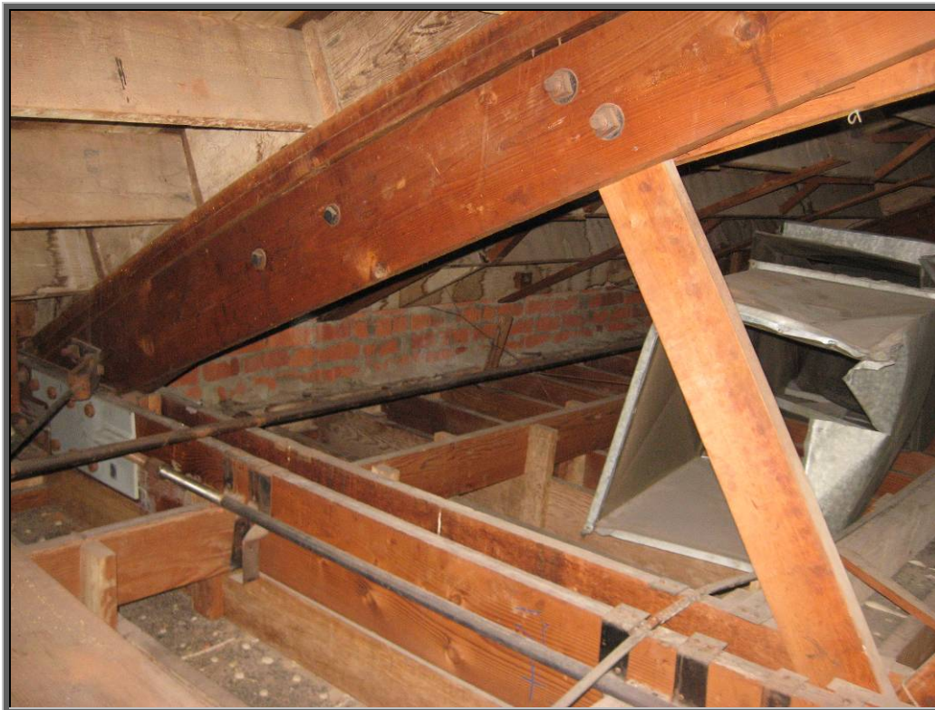
Photo 5: Typical strengthened bowstring truss.
