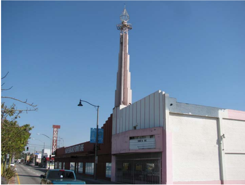
1. West elevation of the theater building looking north.
