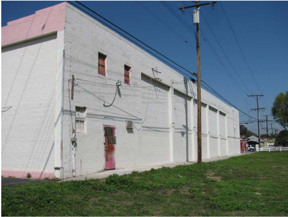
6. East elevation looking north.
