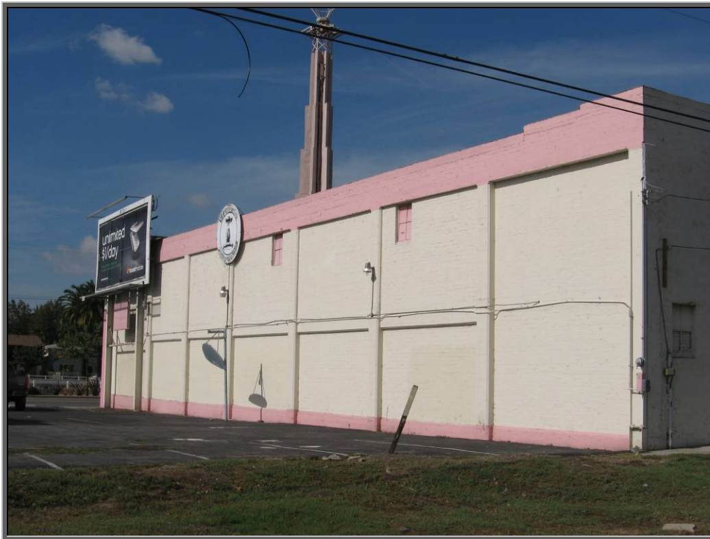
Photo 2: Brick infilled concrete frame at south elevation.
