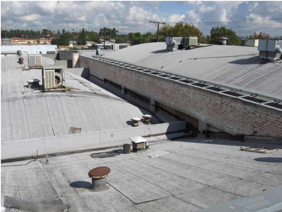
26. View of the different roof areas.
