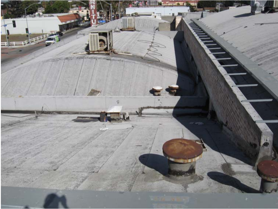
29. Section of the roof over the former furniture store.
