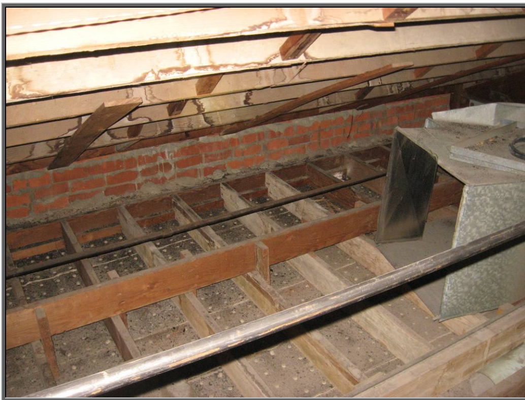
Photo 6: Typical plaster ceiling framing.
