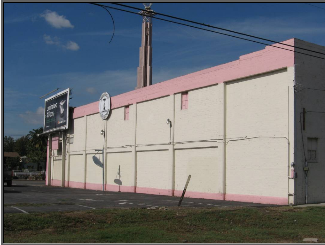
Photo 2: Typical brick infilled concrete frame.
