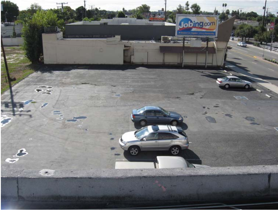
11. Overall view of the parking lot.
