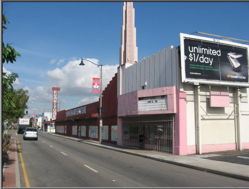
Photo 1: West (Storefront elevation).
