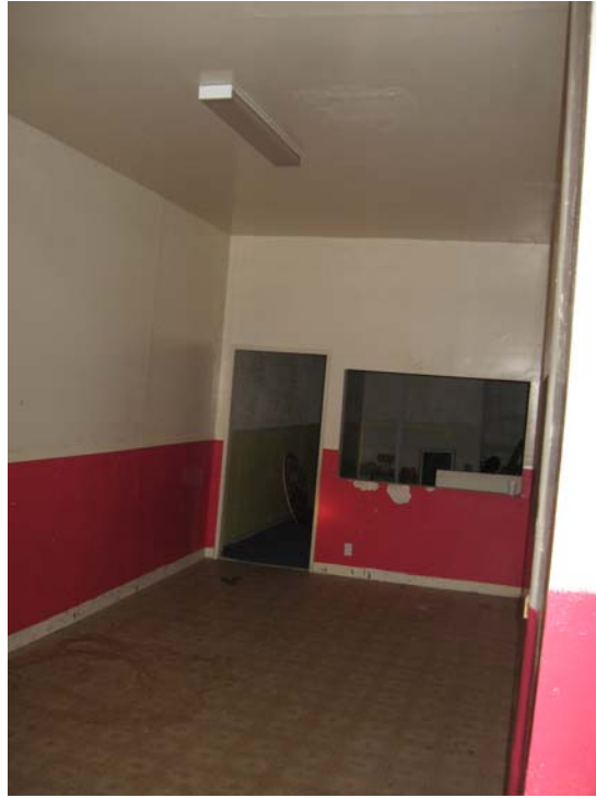
25. Restrooms inside the former church.
