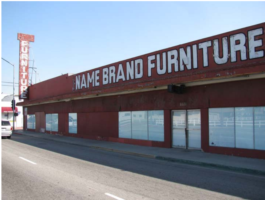
4. West elevation of the Hanson Building.
