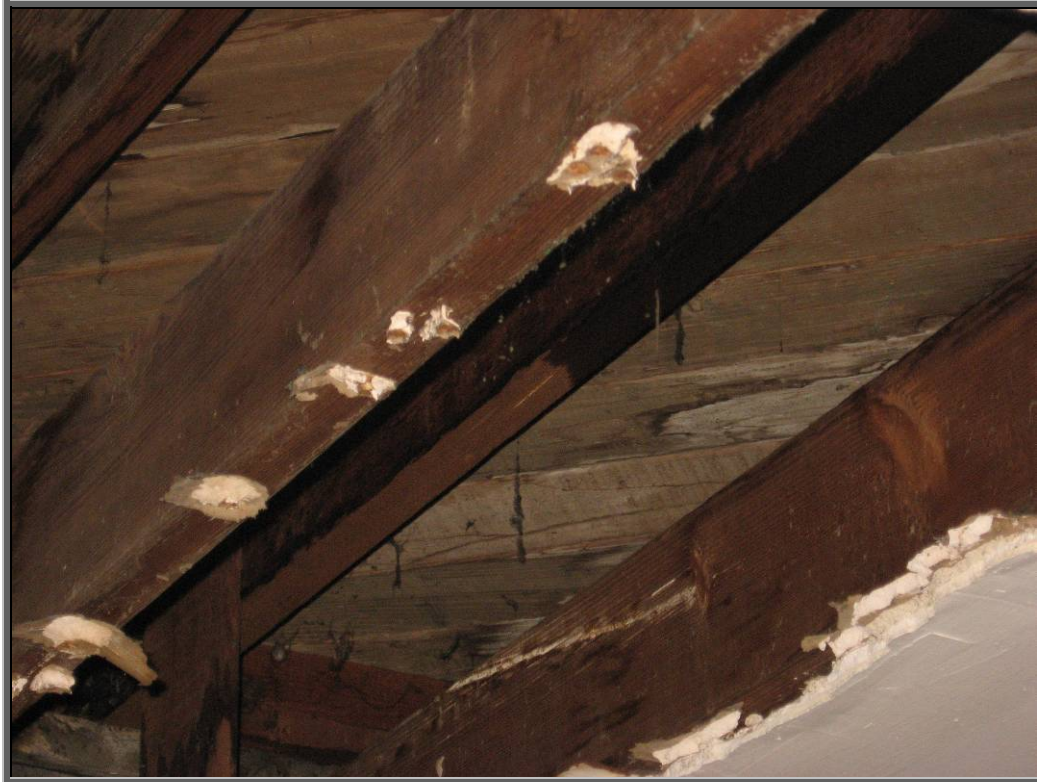
Photo 4: Typical diagonal roof sheathing.
