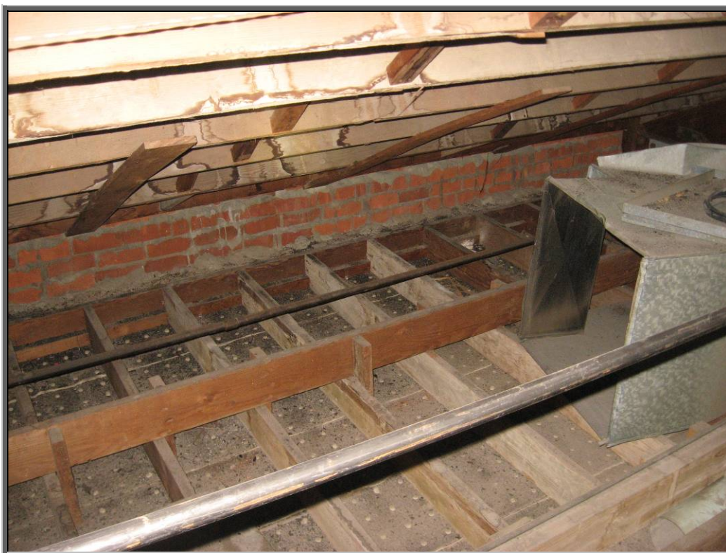
Photo 6: Typical plaster ceiling system.
