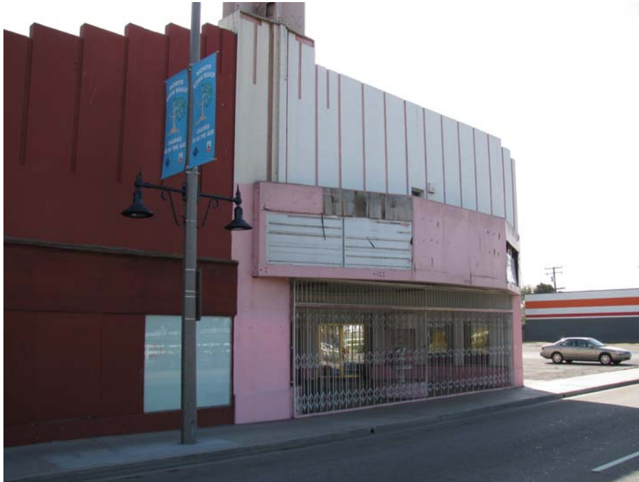
3. West elevation of theater looking south.
