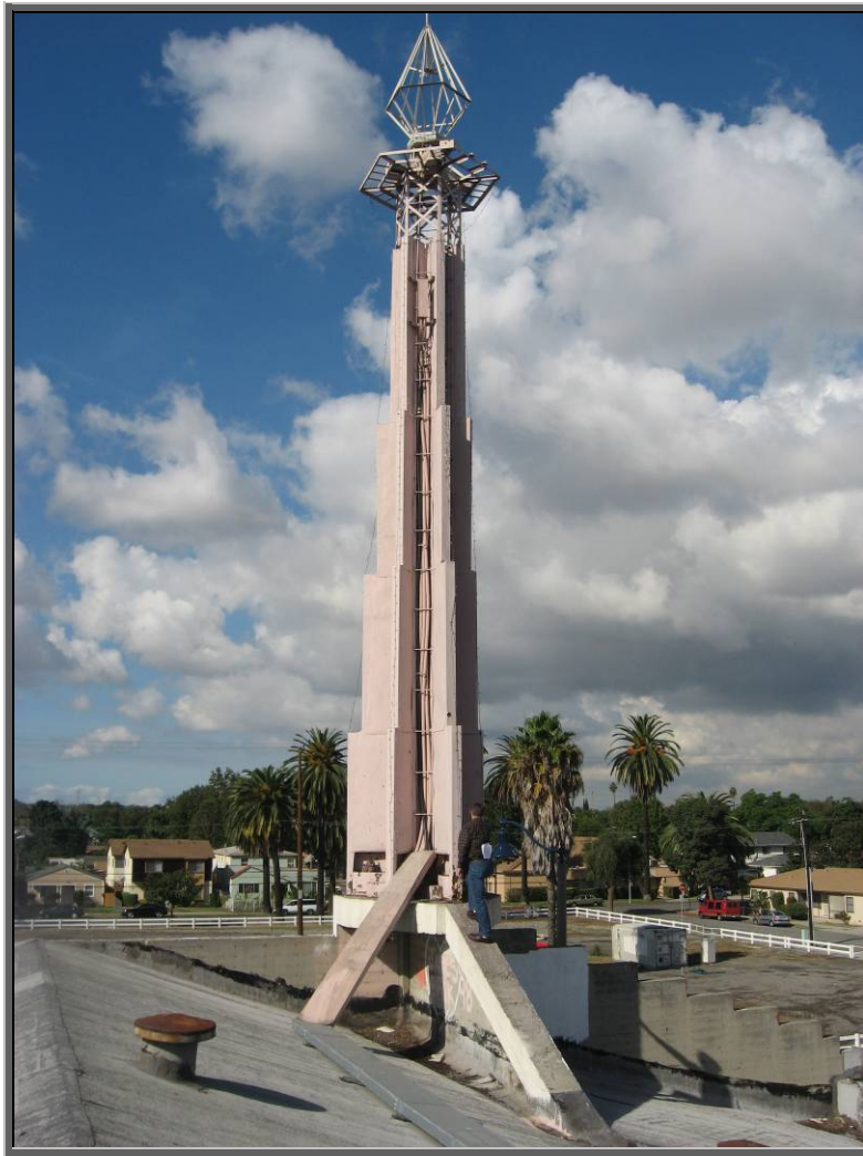
Photo 10: Steel tower spire founded on concrete podium.
