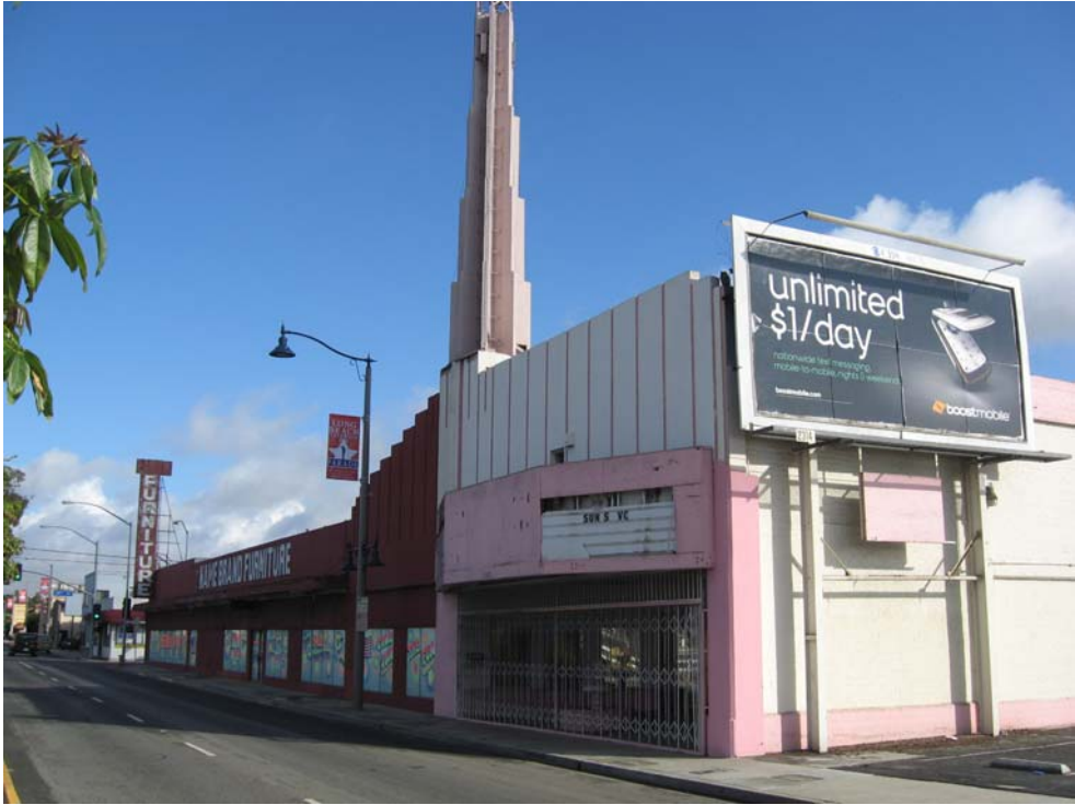
1. Overall view of the property.
