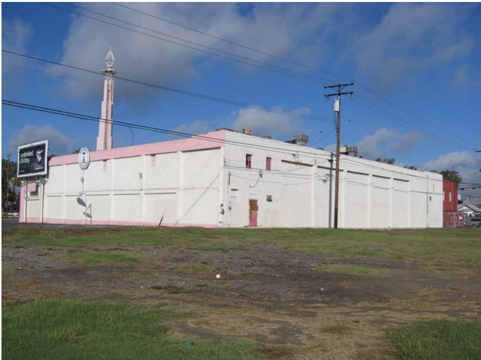
6. South and east elevations.
