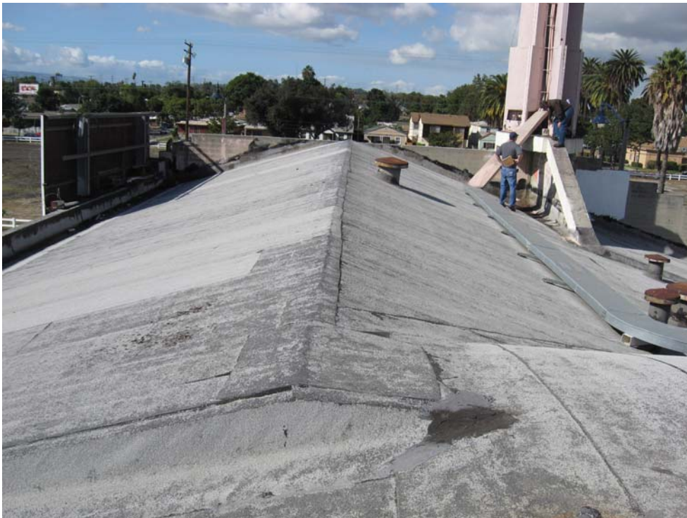
28. Section of the roof over the former church.
