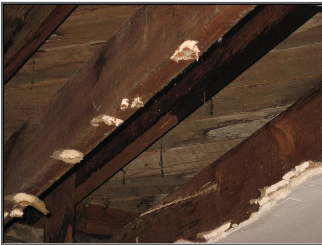
Photo 4: Typical diagonal roof sheathing.
