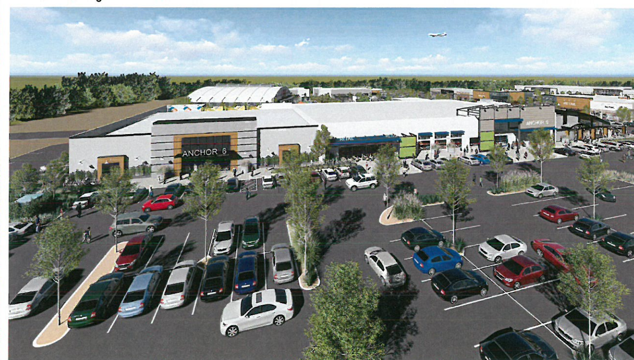
Anchor 5 & 6 & Junior Anchor 1 - East Facade - View from Lakewood Blvd.
