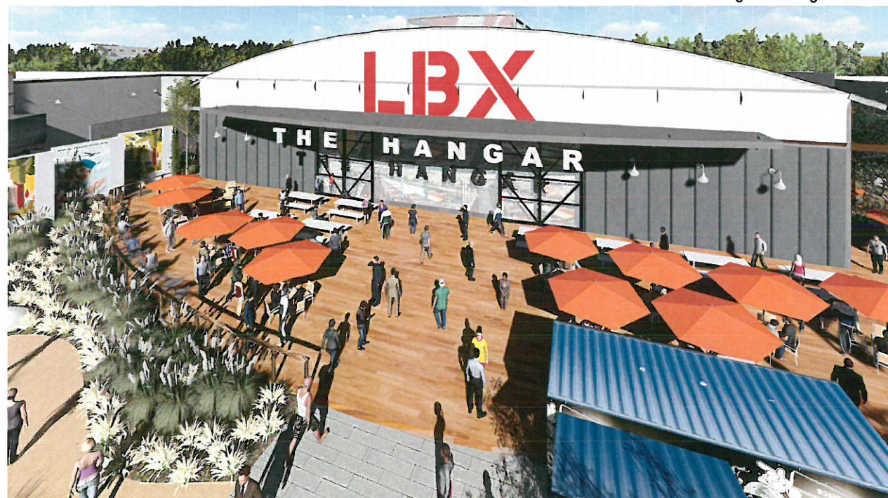
Hangar Building- West Facade - View Looking South-East
