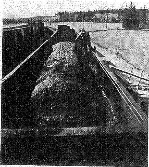
《 PLATE NO.7: HAND APPLICATION OF ASPHALT EMULSION
