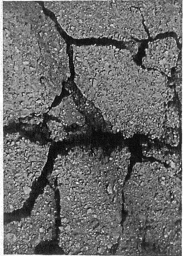
PLATE NO.11: CLOSE-UP SHOWING PENETRATION OF BINDER >
