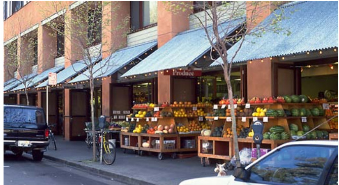
This new storefront building includes bays divided by pilasters that continue through the second story and reinforced by awnings.
