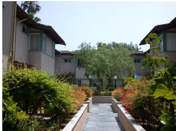
Courtyards over parking can be designed to incorporate landscaping, but some at-grade landscaped areas should be provided to accommodate large trees and landscaped areas that are not behind planter walls.
