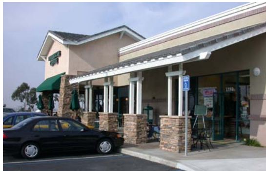
Covered walkway between parking and building entry widened to accommodate outdoor seating.
