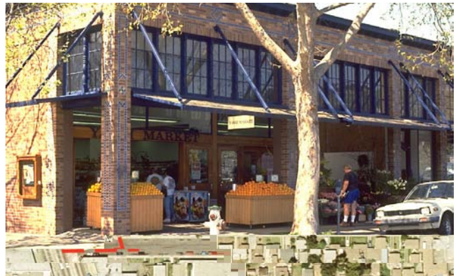
New canopies were added to this older building. Bays are retained and opened to the street.
