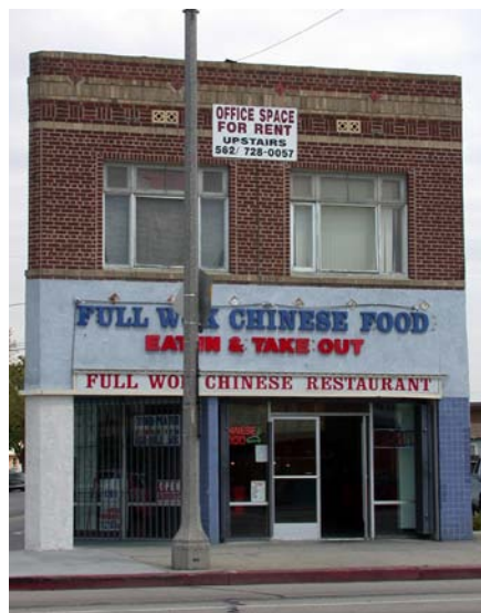
The first-story facade of this masonry building has been stuccoed and tile bulkheads and columns have been removed or covered.
