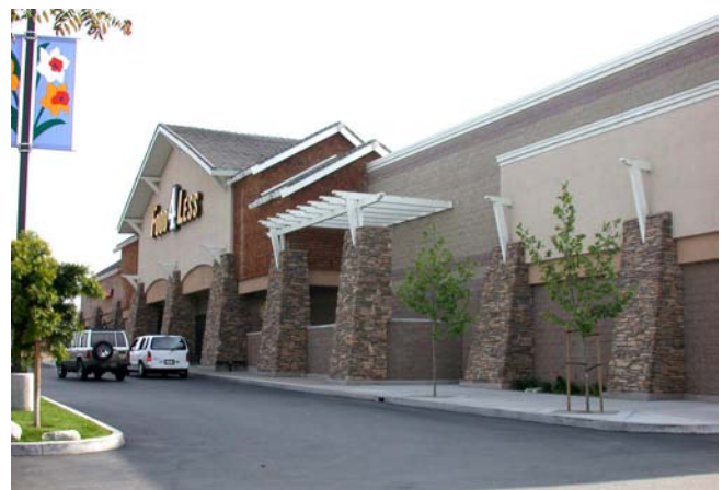
This supermarket building is modulated and articulated by pilasters, a continuous cornice, trellis structures and a central element at the entry.
