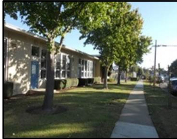
PHOTO 2: School building on E. Ridgewood St. (looking east)
