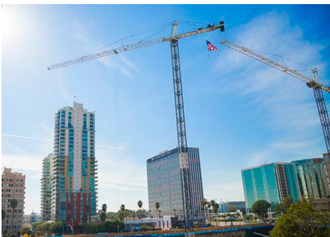
Construction of city hall
