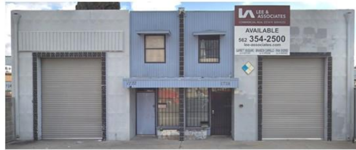
EXISTING WEST FACADE
