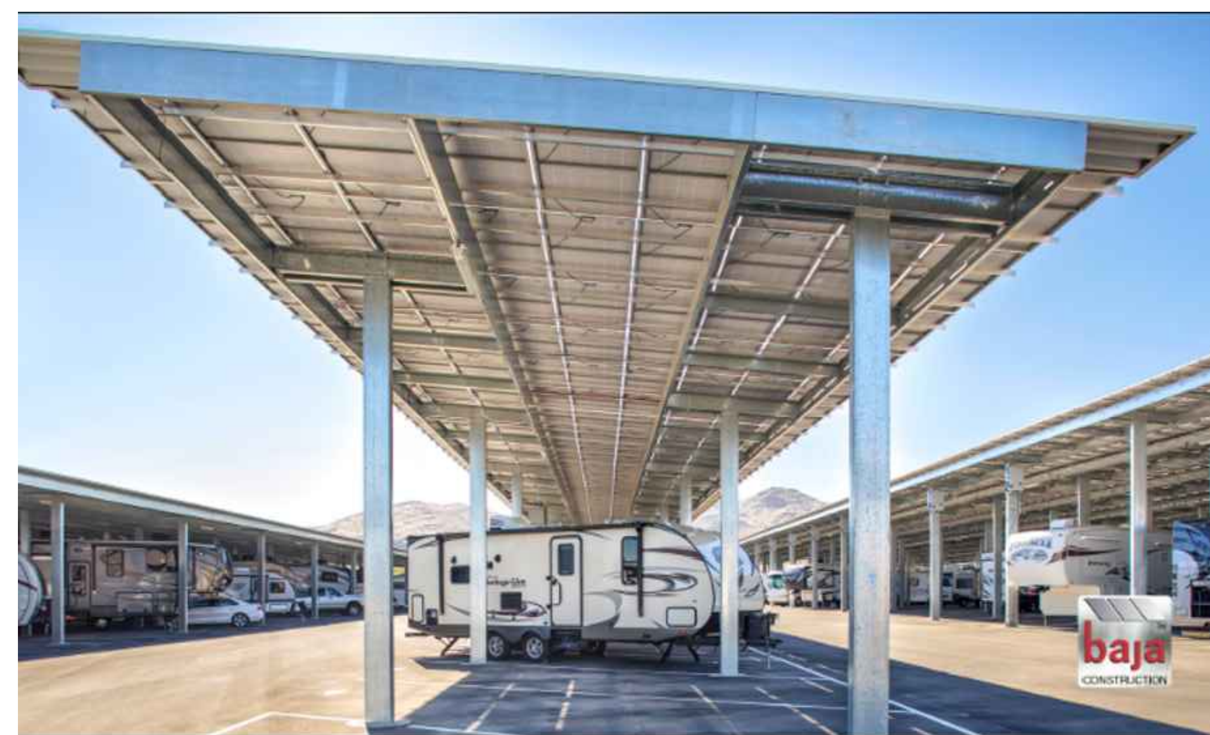
RV PARKING STRUCTURE
