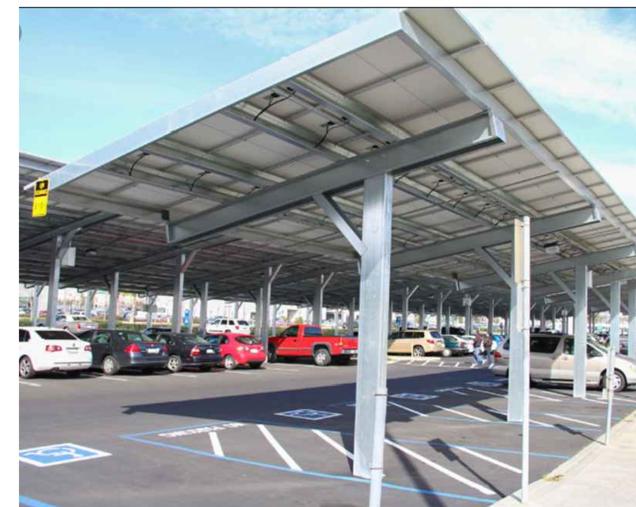
RV PARKING STRUCTURE
