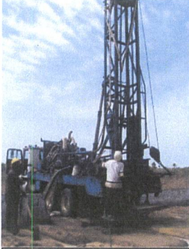
Drilling in Progress
