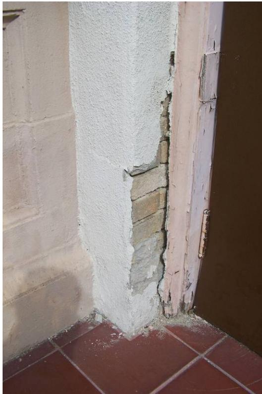
Original Brick Beneath Stucco on West Elevation
