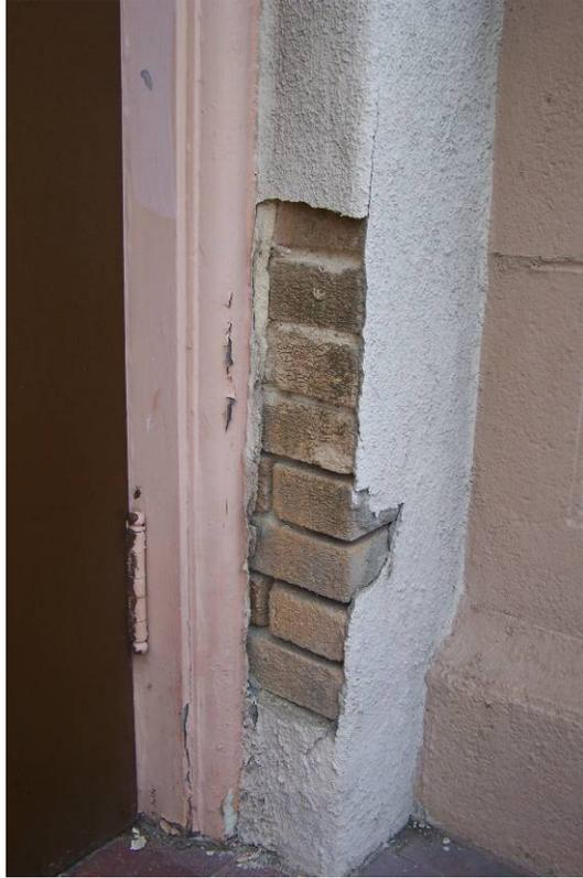
Original Brick Beneath Stucco on West Elevation
