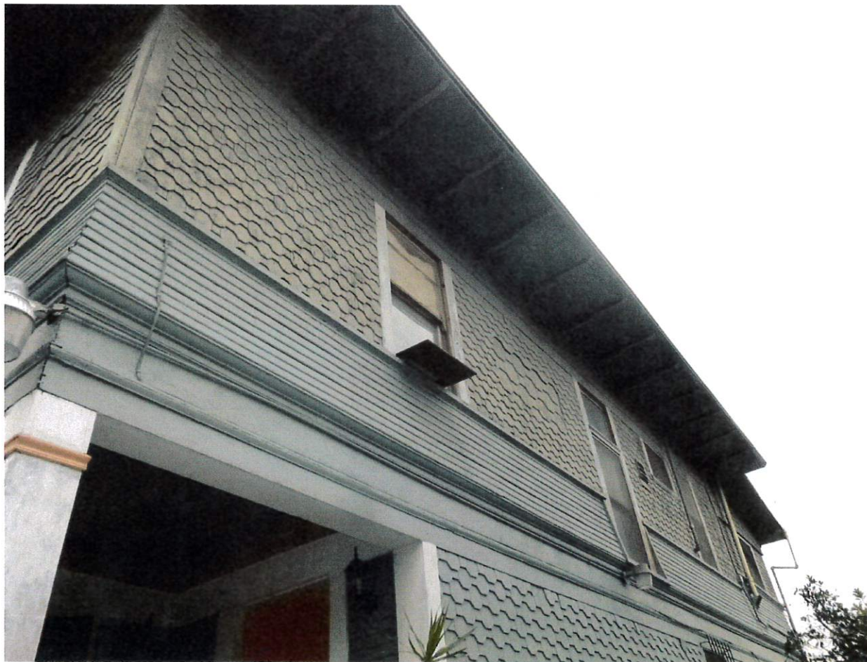
East elevation over the porch, shingled mosaic pattern visible. Sash windows.
