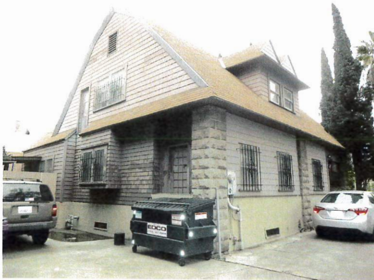
Southwest elevation of 1005 Locust Avenue. Detail of double gabled dormer and 2 nd story exterior door, added in 1977 and currently inaccessible.
