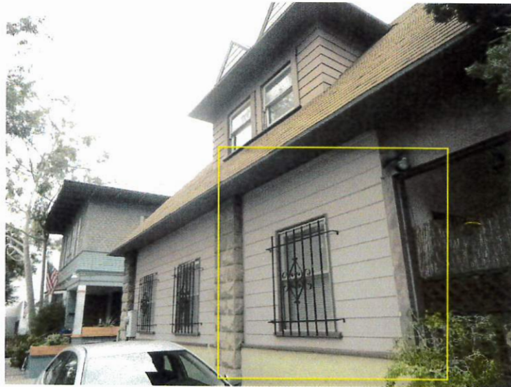
South elevation looking northeast from the corner of 10th and Locust. Detail shows side porch, which has been enclosed.
