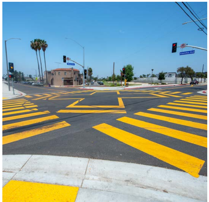
A pedestrian scramble crossing at Alamitos and Walnut Avenues makes crossing the street easier and safer.
