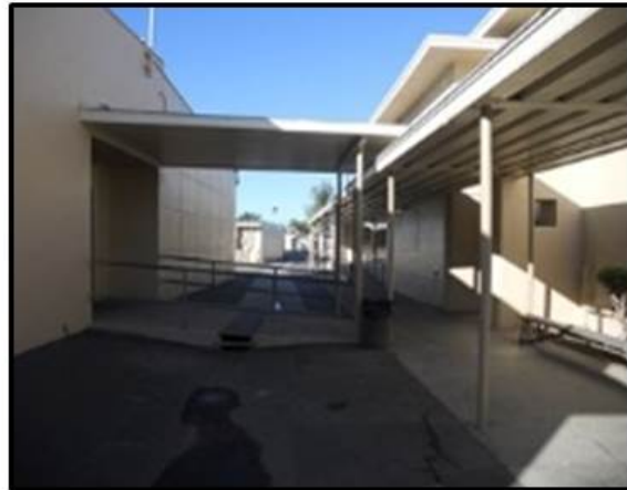
PHOTO 4: Drainage between two northern buildings in walkway (looking west)
