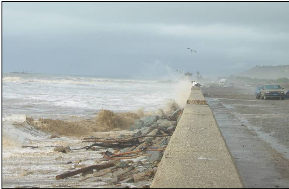
Figure 14. An example of coastal armoring leading to the disappearance of beach
