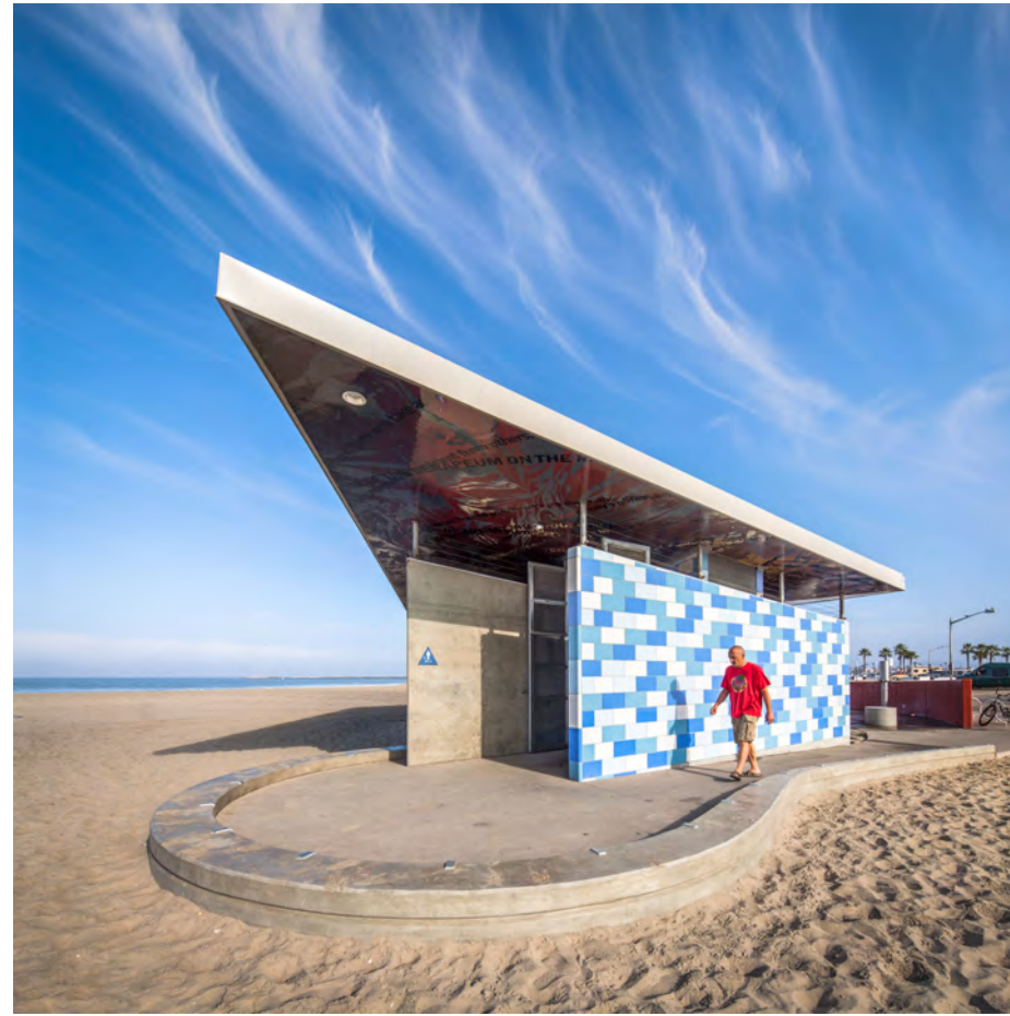
2. OCEAN BEACH COMFORT STATION KEVIN DE FREITAS
