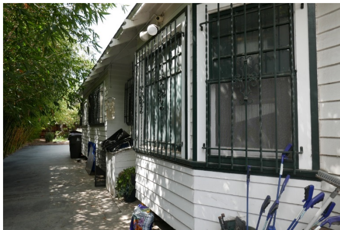
Eastern Façade, 1400 Hellman Street
