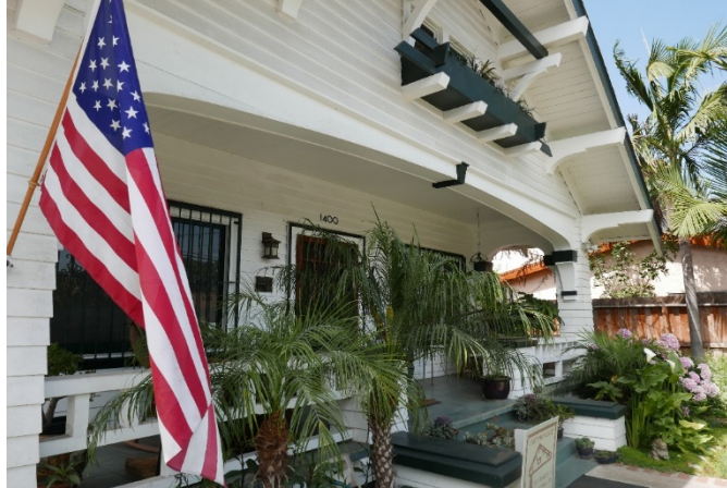
Primary (Northern) Façade, 1400 Hellman Street
