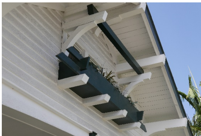
Detail, Primary (Northern) Façade, 1400 Hellman Street
