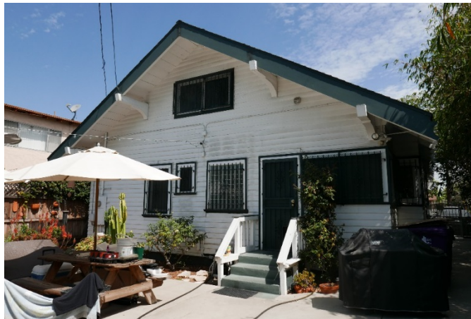
Southern Façade, 1400 Hellman Street
