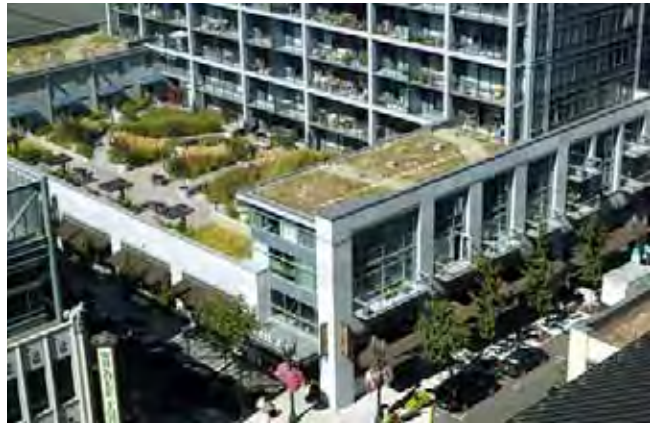
Example of a green roof on the lower floors of a mid-rise building that collects rainwater and provides open space with visual benefits.
