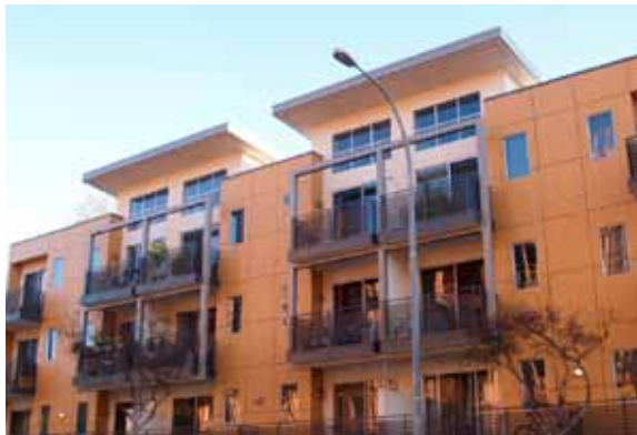
Example of reinforced fiber cement panels integrated in a low-rise residential project.
