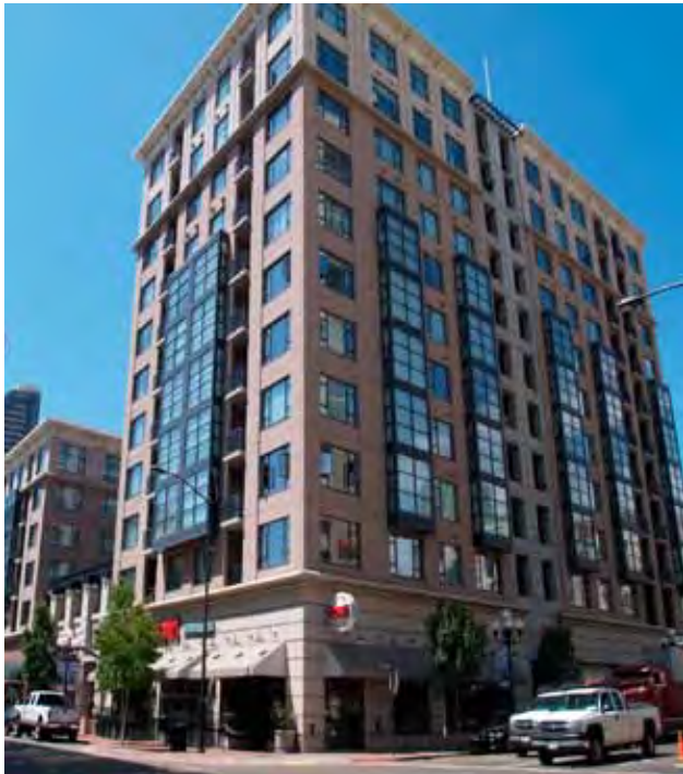
Example of high-quality materials used on a new mid-rise building that exhibits a classic base, middle and top composed of more substantial material and storefront details at the pedestrian level, plus inset balconies and a variety of window types.
