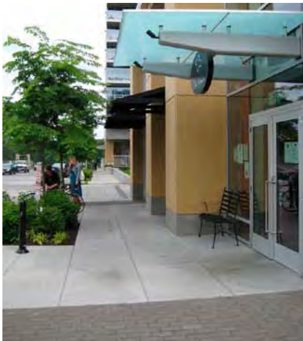
Standard grey concrete sidewalks may be complemented by pavers of a similar color (above) or sawcut in a diagonal pattern (right) to add visual interest.
