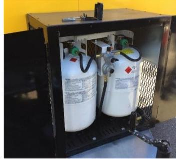
**Propane Tanks w/ Dual regulator**
