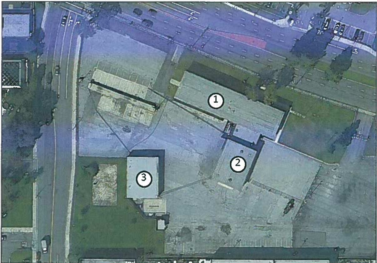
Figure 2: Components of the property include: 1.) Schroeder Hall administration center; 2.) Schroeder Hall assembly hall; 3.) OMS building. Source: Google Maps.
