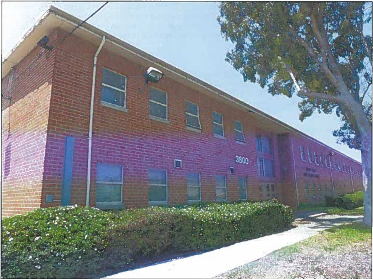
Figure 3: Schroeder Hall, north elevation, administration center. Source: GPA, May 2013.
