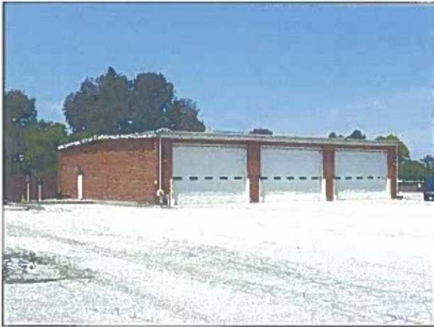
Figure 8: OMS, east and south elevations. Source: GPA, May 2013
