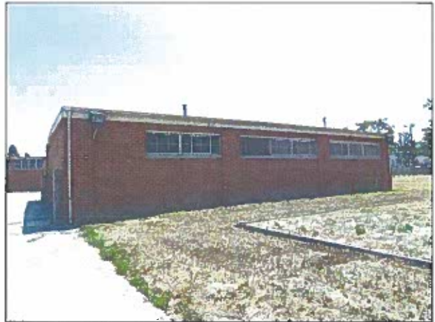
Figure 9: OMS, west elevation. Source: GPA, May 2013
