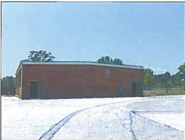
Figure 10: OMS, north elevation. Source: GPA, May 2013
