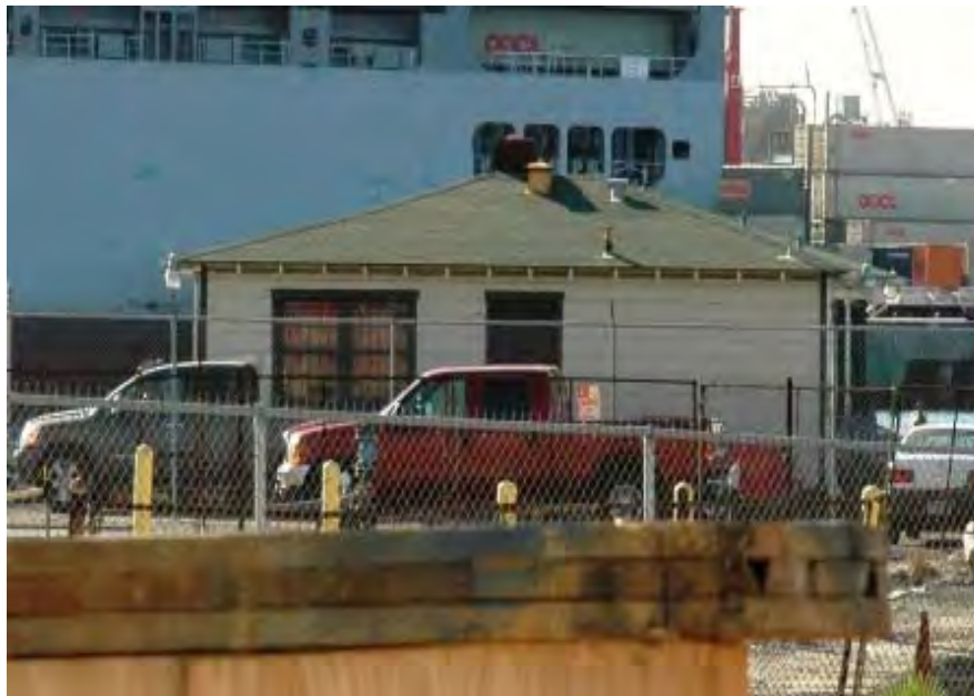
Smoke House/Office E23
