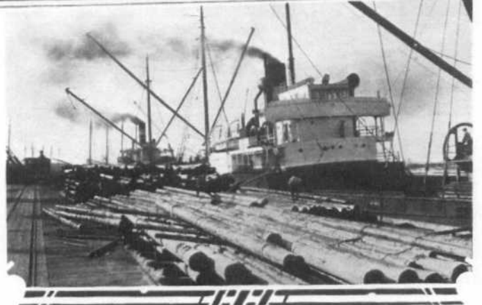
Loading Creosoted Piling at Plant of J. H. Baxter & Co.
