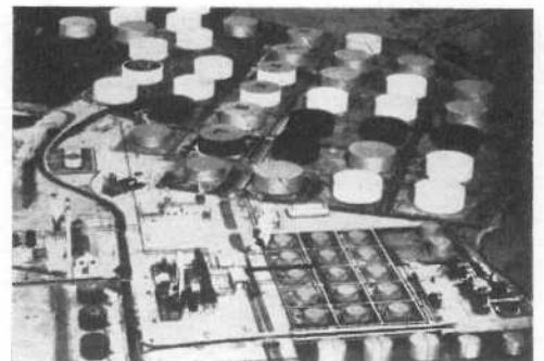
OIL STORAGE TANK FARM
