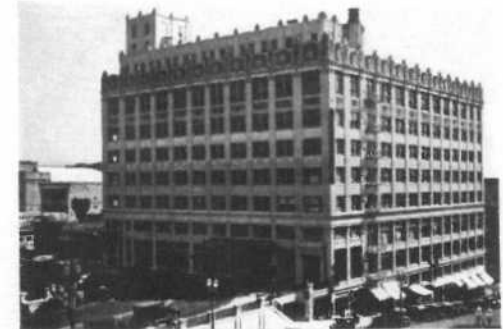
JERGIN'S TRUST OFFICE BUILDING (Home of Municipal and County Courts)
