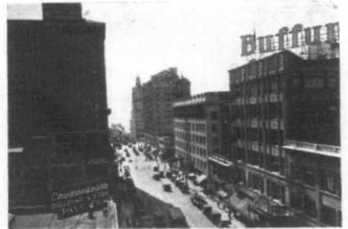
BUFFUMS' DEPARTMENT STORE (Pine Avenue, Looking South)
