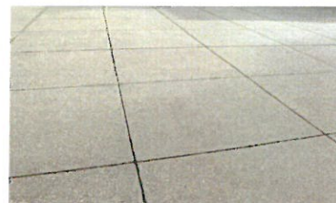
ENHANCED CONCRETE PAVING COLOR: SCOFIELD 'ADOBE TAN' C-21 SAWCUT SCORE PATTERN: 5' X 5' DIAGONAL
