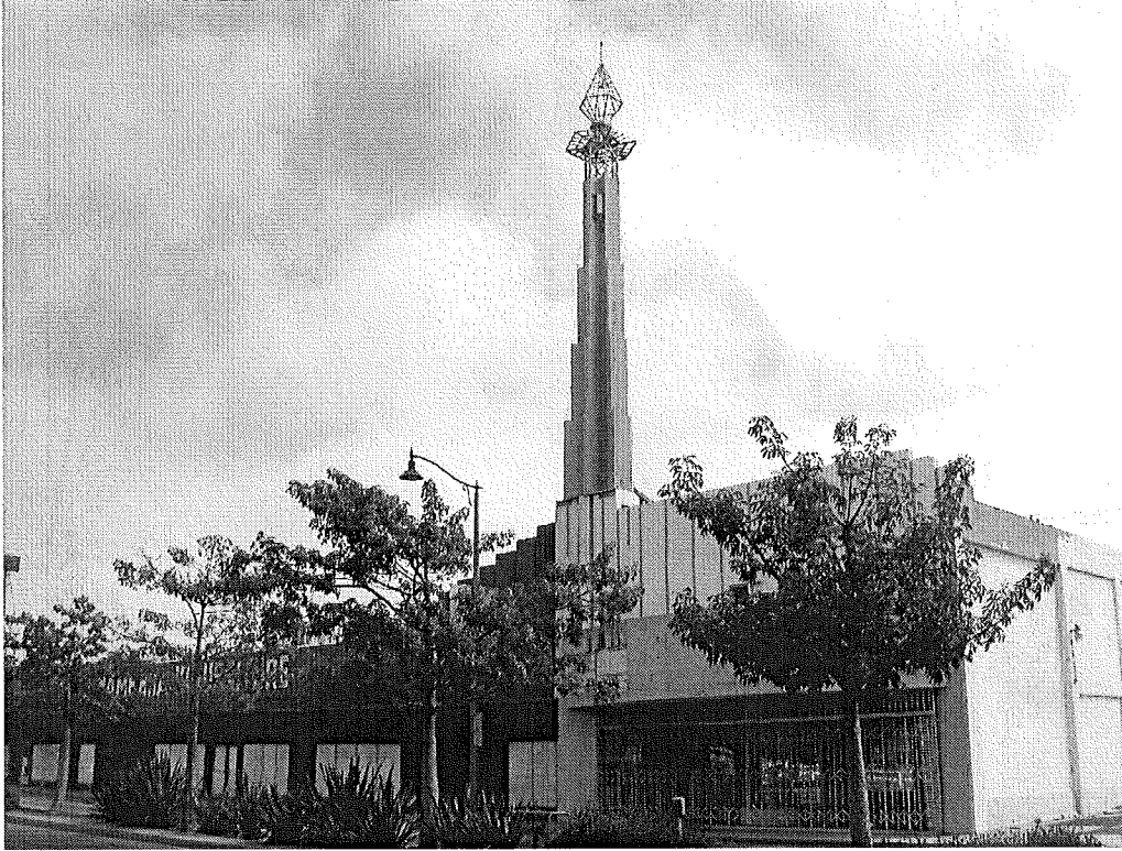
Subject Property – Cell Tower located on structure at 5870-5874 Atlantic Avenue
