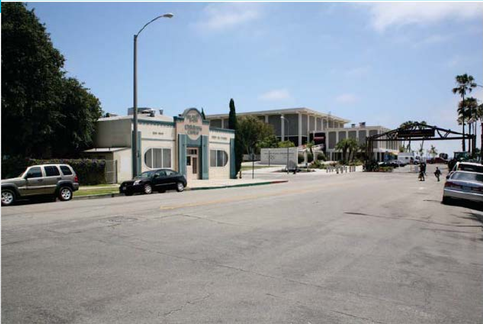
Key View 1: Before View facing south at intersection of Termino/Midway
