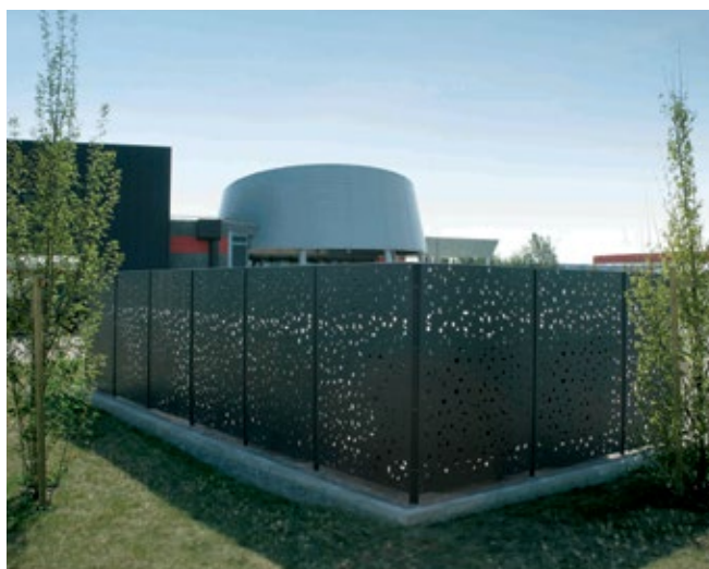
Metal screen used to screen utility area. Source: idmetalco.com
