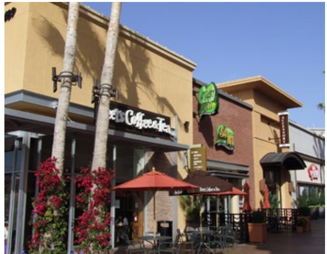
Buildings face pedestrian pathway.
