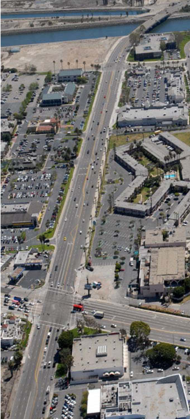
PCH looking south. Existing commercial and hotel uses on either side of the street are the SEASP's primary opportunities to accommodate land use changes that can respond to future growth in the area and also to create a pedestrian-friendly activity center as described in the SEASP Vision. At the top of the photo, the bridge over the San Gabriel River that extends into Seal Beach serves as a visual and physical gateway into Long Beach and the SEASP area.
