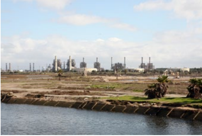
Existing view corridor across the Los Cerritos Channel and Wetlands.
