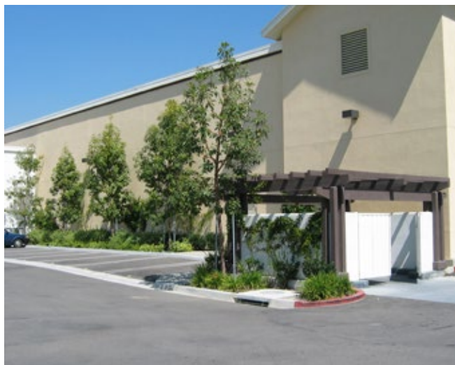
Pergola used to screen utility area.
