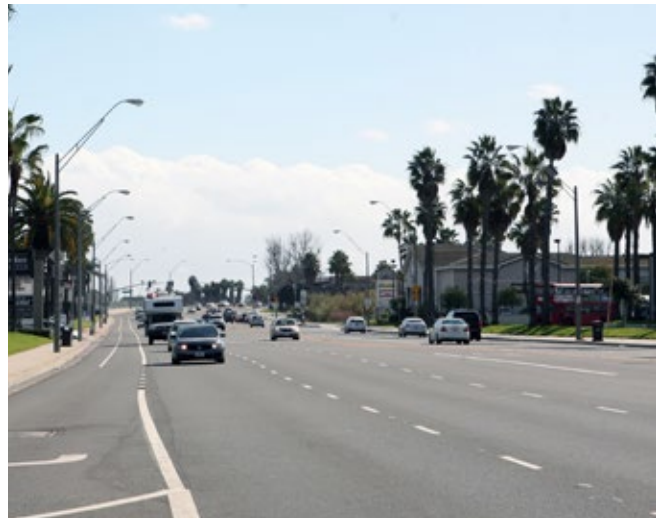
Much of the supporting infrastructure for the SEASP area runs under major thoroughfares such as 2nd Street, Pacific Coast Highway, and 7th Street.
