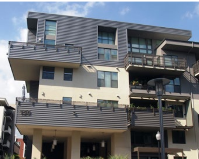
Balconies that shield visibility of personal items from public view.
