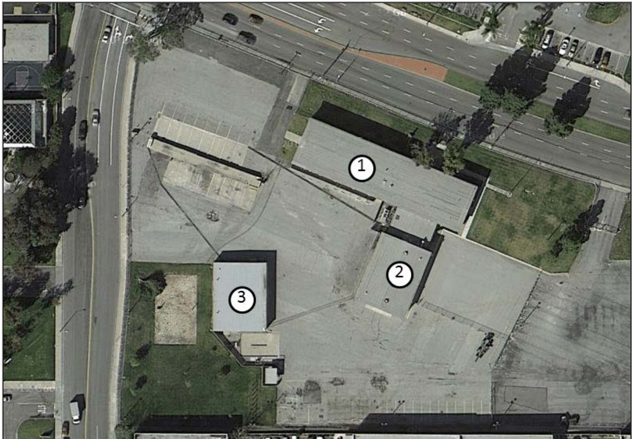
Figure 2: Components of the property include: 1.) Schroeder Hall administration center; 2.) Schroeder Hall assembly hall; 3.) OMS building. Source: Google Maps.
