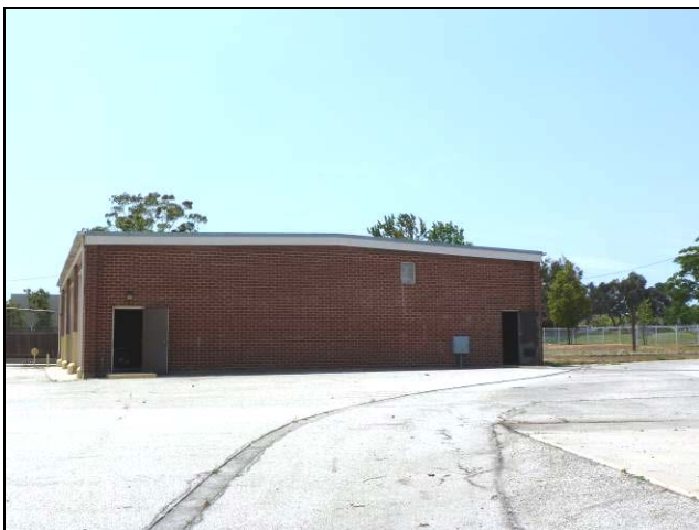
Figure 10: OMS, north elevation. Source: GPA, May 2013
