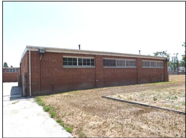
Figure 9: OMS, west elevation. Source: GPA, May 2013
