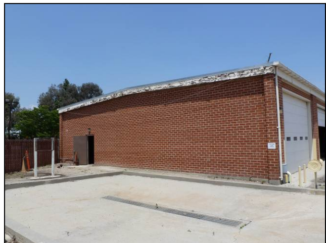
Figure 11: OMS, south elevation. Source: GPA, May 2013
