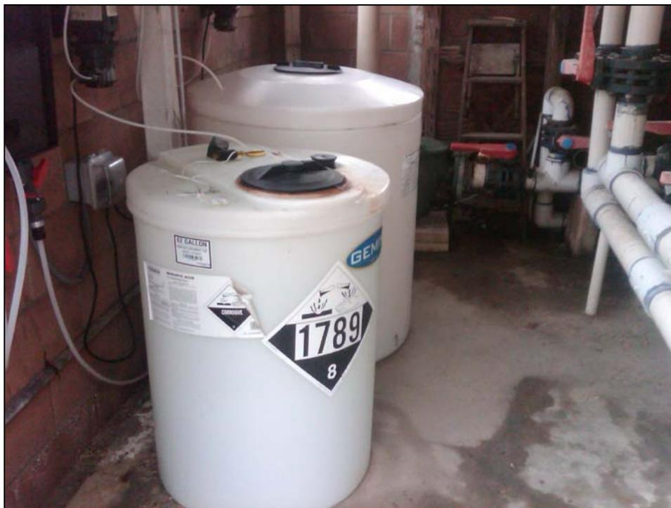
Photograph 6. Interior photograph of the pool pump house enclosure showing the chlorine and muriatic acid tanks for swimming pool maintenance.
