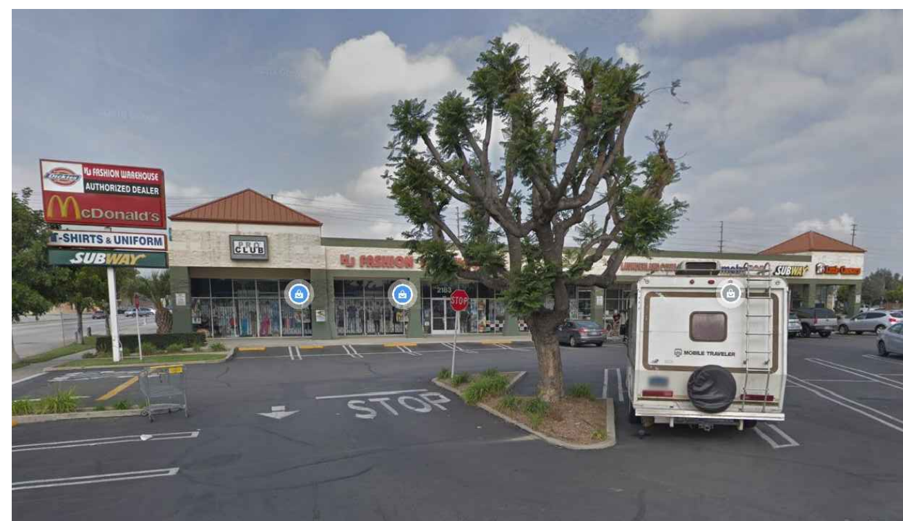
7 EAST VIEW BUILDING B
