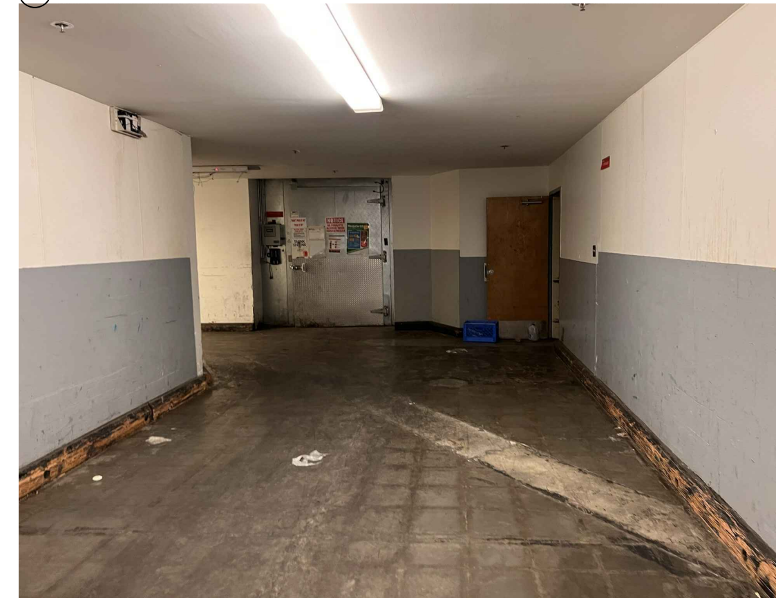
11 INTERIOR HALLWAY VIEW
