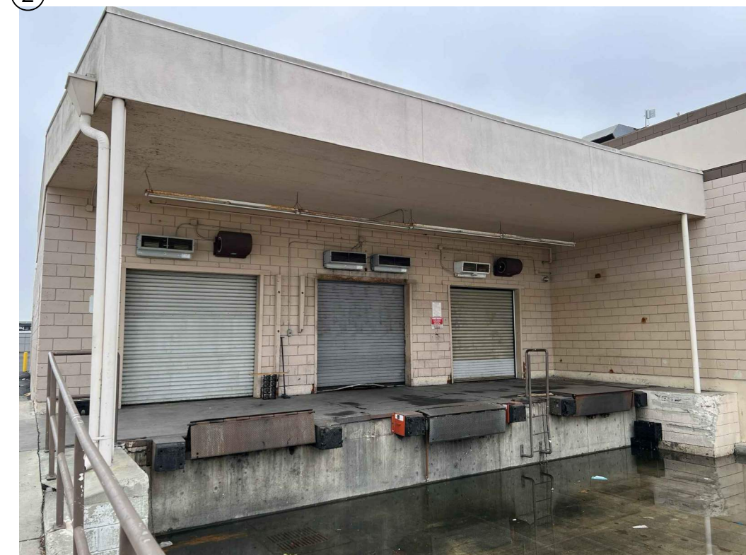
3 LOADING DOCK NORTH SIDE
