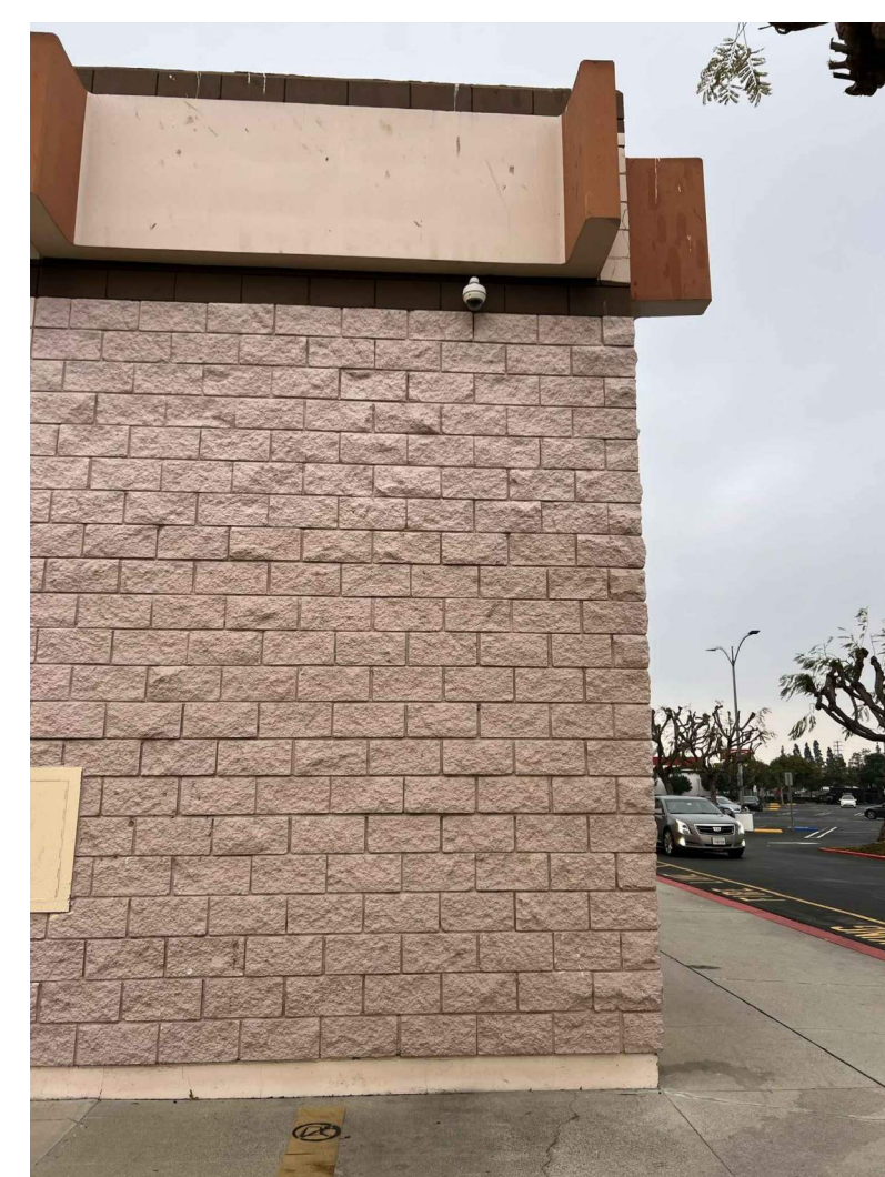
5 SOUTHWEST CORNER OF EXISTING BUILDING
