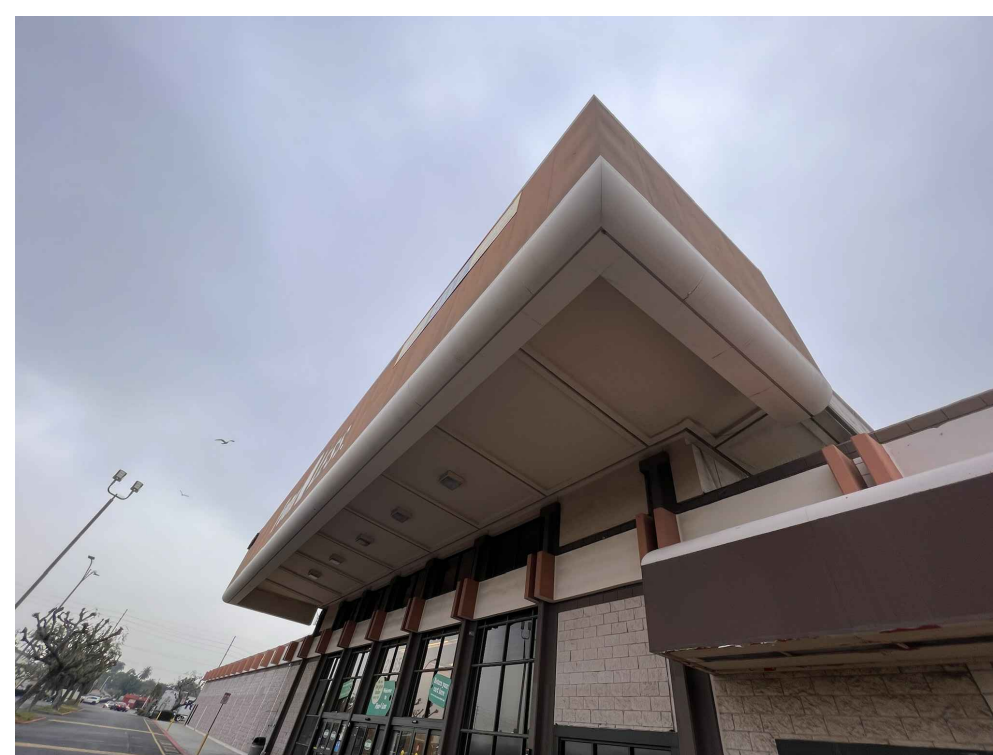
6 MAIN ENTRANCE SOUTH VIEW
