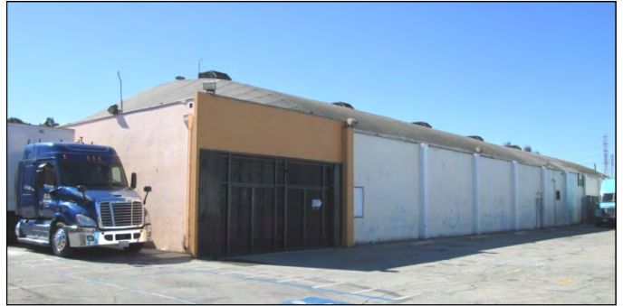
Detail of 6845 Atlantic Avenue, east and north elevations, view to the southwest.
