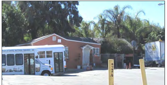
Residence located near the southern property line behind 6845 Atlantic Avenue, view to the south.
