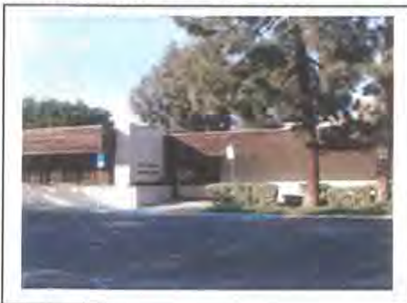
North Facilities Center
