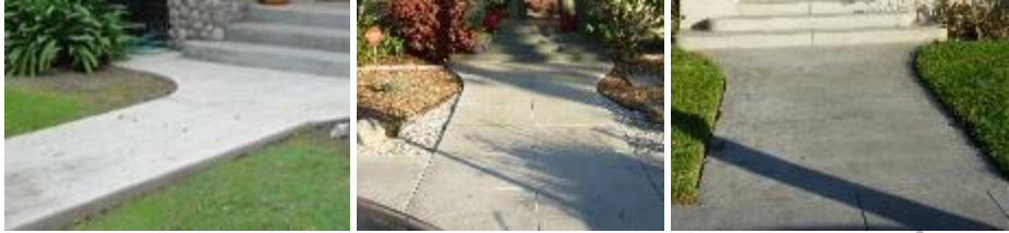
Caption: Walkways in the Bluff Heights Historic District are primarily concrete with scored joints; many “bow” out to meet the edges of the porch steps.
