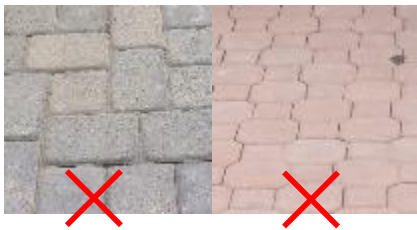
Caption: Contemporary concrete pavers are not appropriate for use in the Bluff Heights Historic District.
