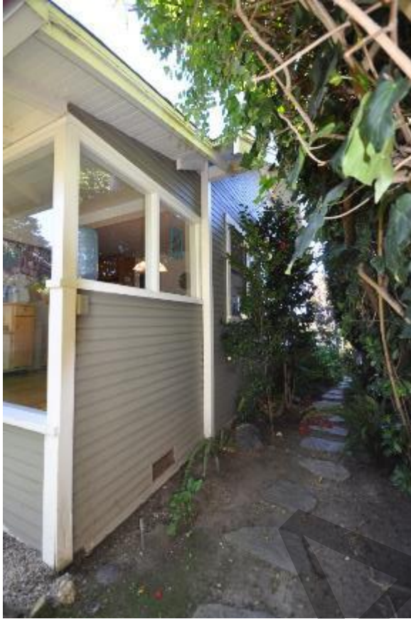
Caption: This compatible addition is differentiated from the main house by fixed single-light windows and a vertical strip of trim.
