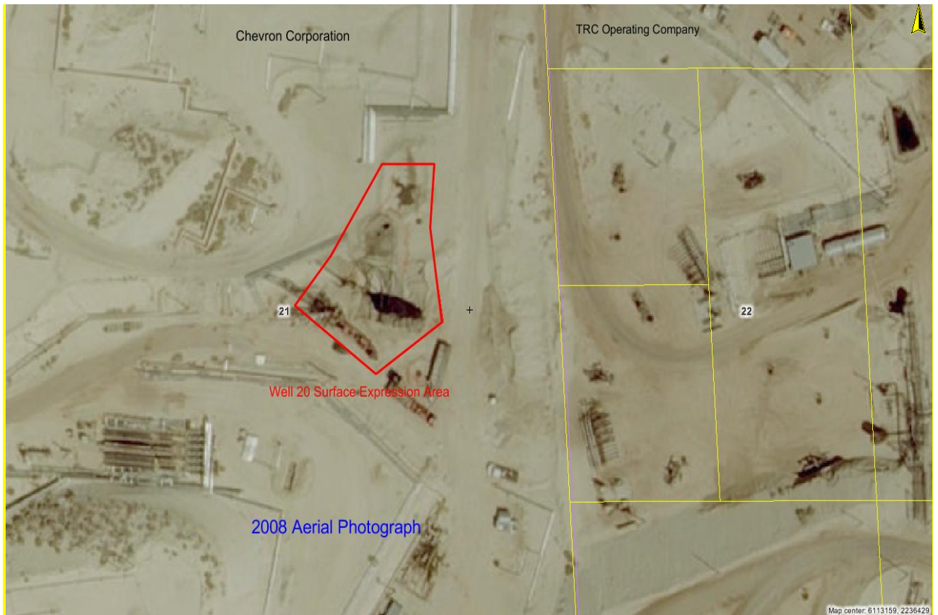
Aerial Photograph 1 – 2008 aerial view of the Chevron Well 20 surface expression area, showing the surface expression containment pit as well as other surface expressions in the immediate vicinity.
