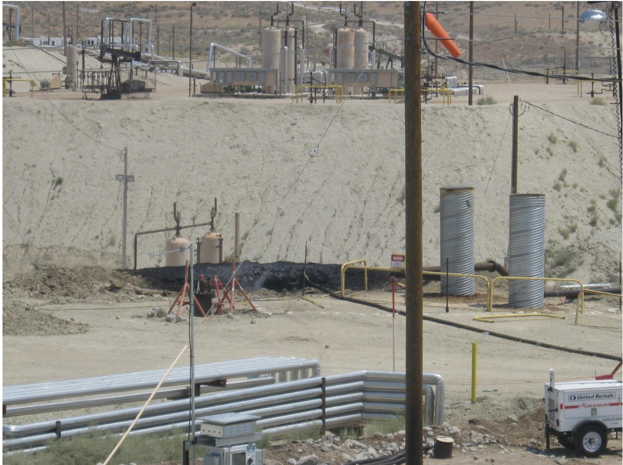
Photograph 15 – View of the Chevron accident location on July 7, 2011. The release of fluid and steam to surface had increased significantly since the June 21 accident, as well as the enlargement of the associated crater.
