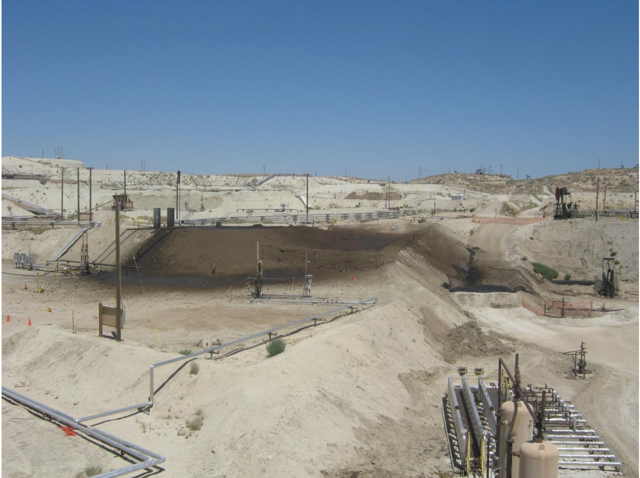
Photograph 19 – View of the Chevron Well 20 and the nearby TRC surface expression areas, on August 5, 2011. The eruption expelling rocks, water and oil occurred sometime during the night of August 4.
