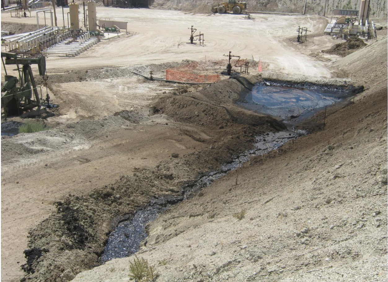
Photograph 22 – View of the two new TRC surface expressions that became active on August 3. They are located at the top and bottom of the stream of fluid. The bermed pit was put in place after the reactivation of a surface expression at that location on June 27.
