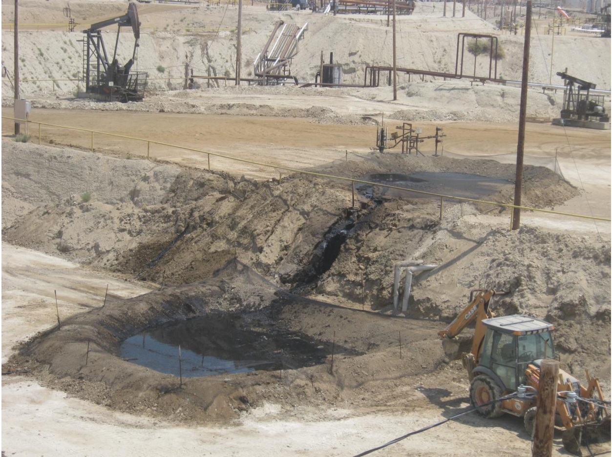
Photograph 17 – View of surface expression on TRC’s “Bull” lease, July 7, 2011. An increase in the crater diameter on the upper terrace and deeper erosion of the terrace slope was noted. Approximately 100 bbls/day of fluid was being removed from the containment berm on the lower terrace.
