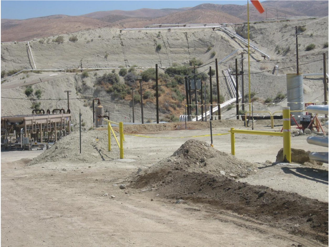
Photograph No. 10 - View of the accident site on the upper terrace overlooking the surface equipment of the subsurface containment structure and the remediated surface expression on June 21, 2011. Well K210 is located on the far right of the picture. The accident spot is 15 feet to 20 feet to the left of the yellow wind sock pole, at the base of the berm. The reddish discoloration of the bermed soil at the accident site, and the future location of the crater, is of interest and may be an early indication of steam migrating to the surface.
