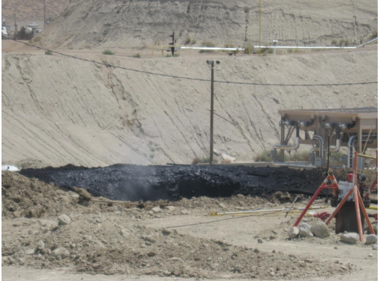
Photograph 16 – View of Chevron accident site on July 7, 2011. The Crater is approximately 10' wide , intermittently expelling oil and water onto the surrounding ground.
