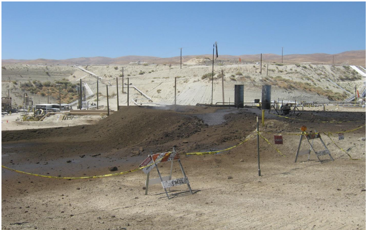
Photographs 20 and 21 – Views on August 5 of the material; water, oil and rocks, expelled from the crater during the night of August 4.
