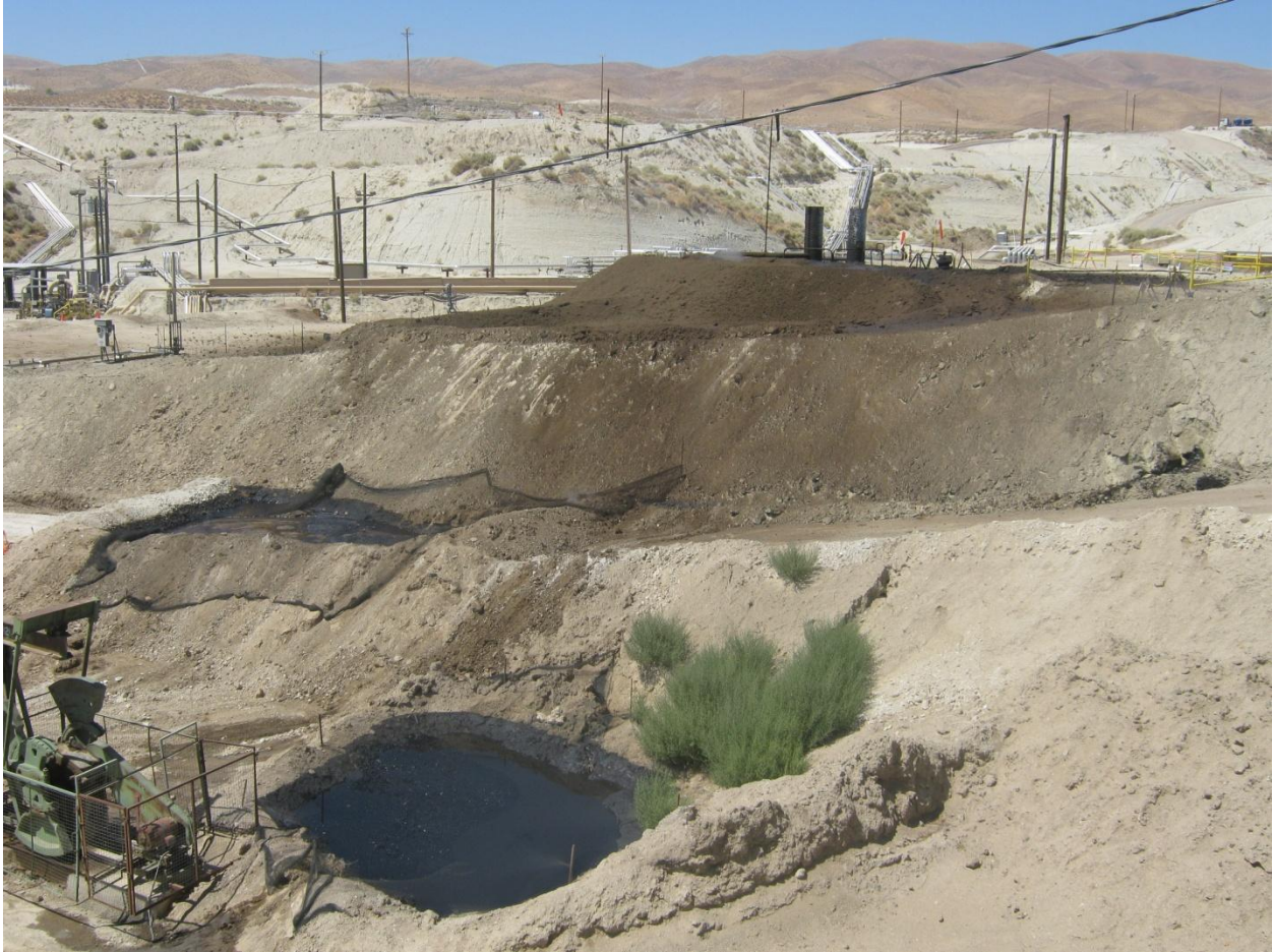
Photograph 23 – View of the eastern extent of the crater eruption onto TRC property and the two new TRC surface expressions located at the base of the oil stained slope.
