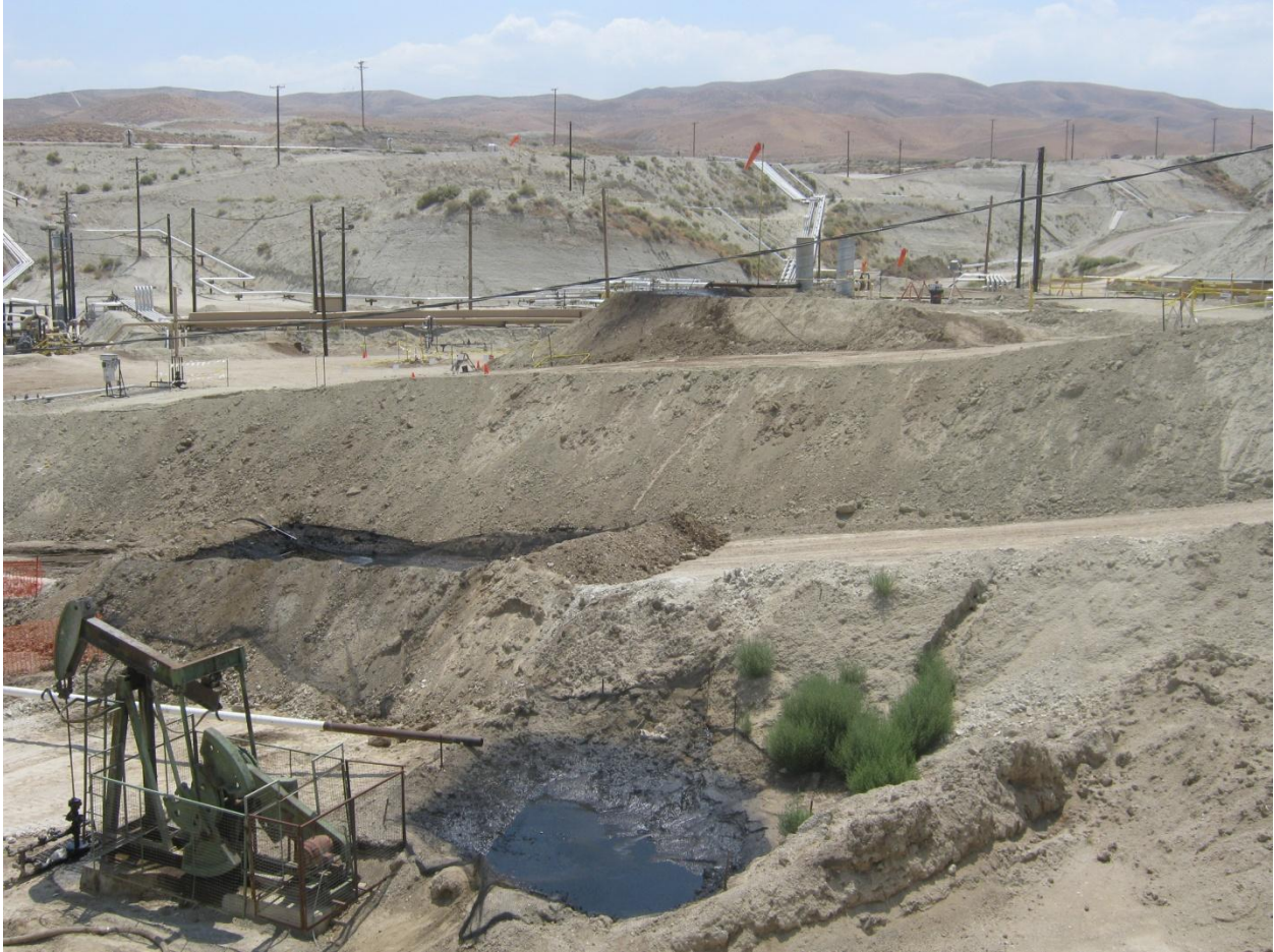
Photograph 18 – View of the TRC reactivated surface expression to the east of the Chevron accident site on July 7, 2011. The TRC reactivated surface expression is at the base of the slope that is essentially the boundary between TRC and Chevron. The crater near the accident site is in the distance with steam rising and oil staining along the terrace slope from fluid recently expelled.
