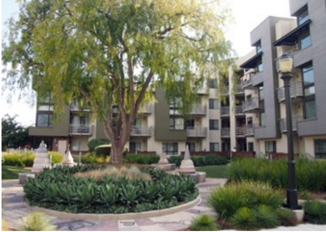
A courtyard fronted by doors, windows, and balconies that provides an interesting gathering space.
