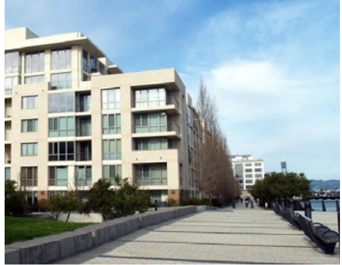
Stepbacks make building heights less imposing and create variation in building massing.
