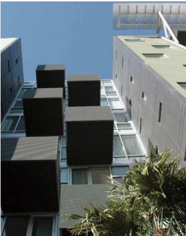
Balconies and overhangs can be used to block the view of glass from birds.
