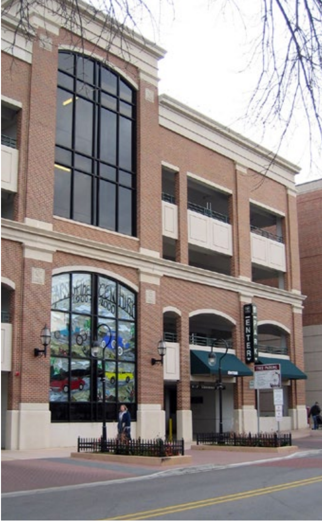
Entrance to a parking structure.
