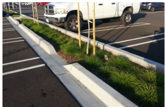
A bioswale in a parking lot can help to reduce stormwater runoff.
