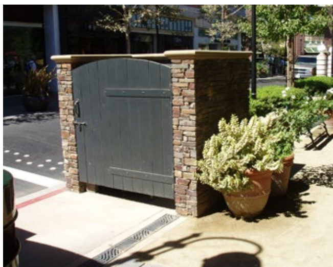
Brick and wood screen for utility area.
