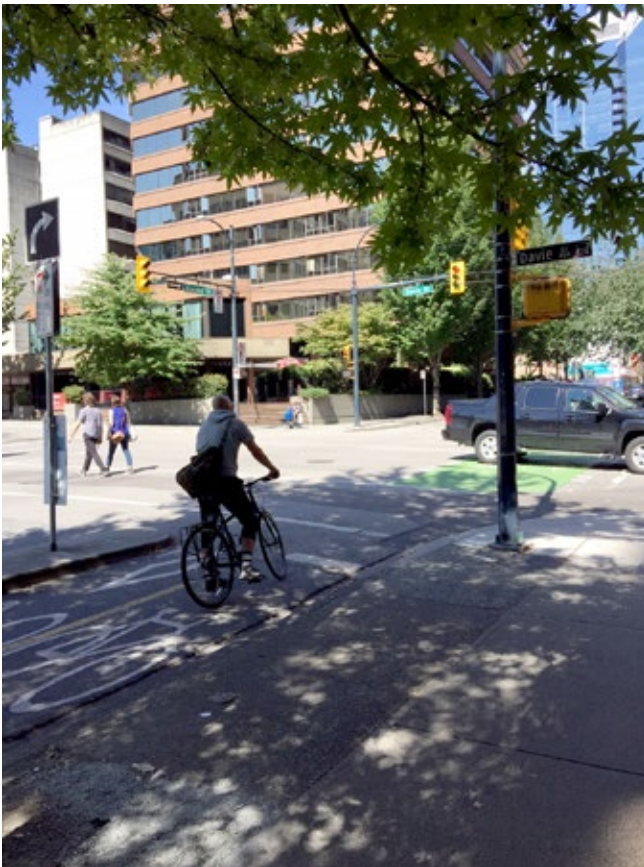
A separated bike lane known as a cycle track provides a safe lane of travel for bicyclists.
