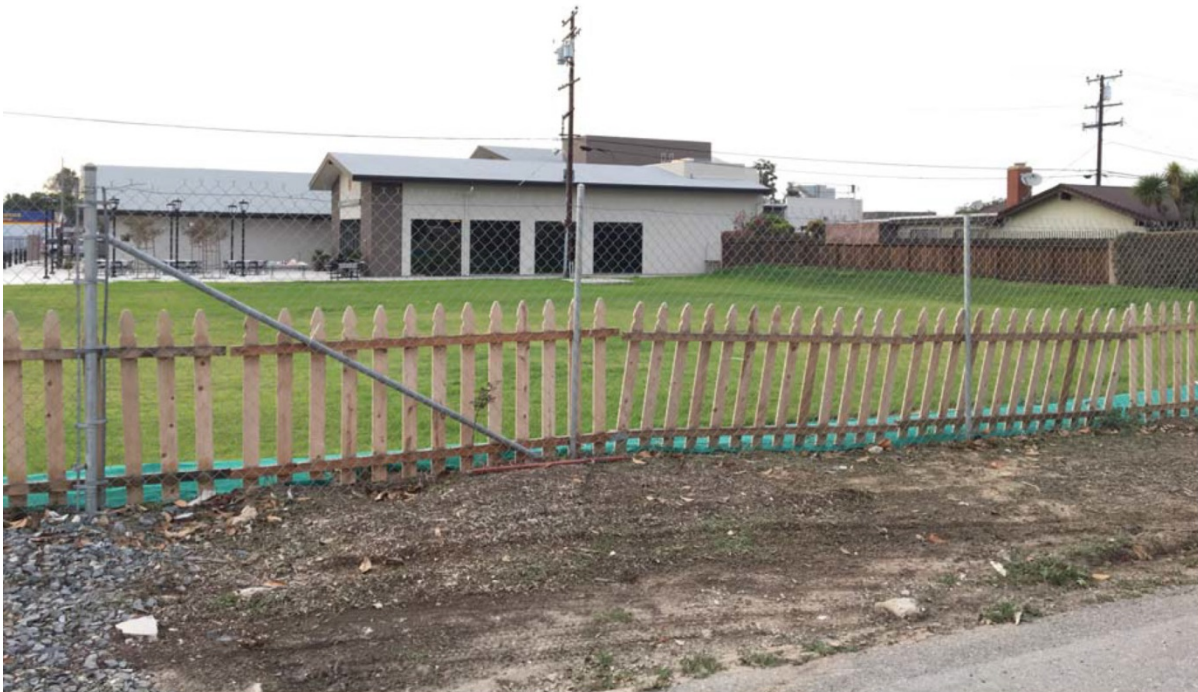
Photo 2: Location of proposed gymnasium as viewed from Elm Avenue, looking west.
