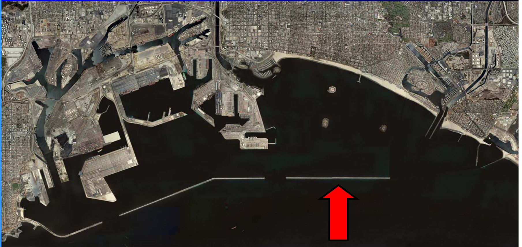
Long Beach Breakwater
