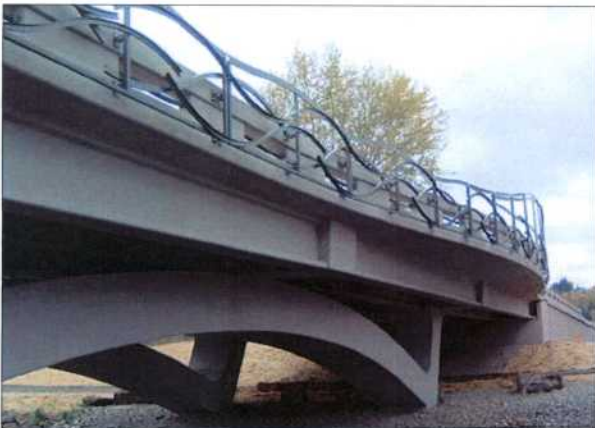
River Crossing, King County, WA
