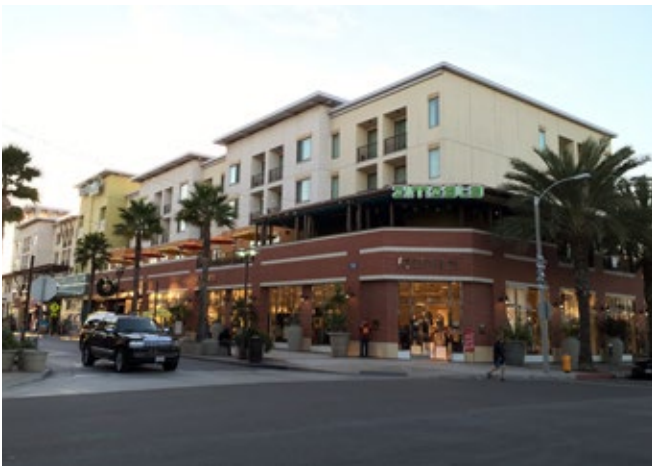
Example of a mixed-use building that provides an active street front and a setback design to upper floors with residential uses.
