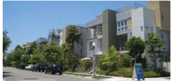
Multifamily Residential – Low: 3-story townhomes.
