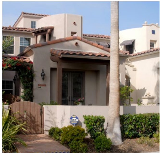
Variation in rooftop design can add interest to a building.
