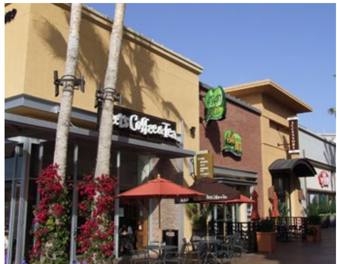
Buildings face pedestrian pathway.
