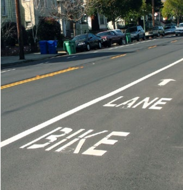
A Class II bike lane provides a delineated right-of-way assigned to bicyclists.
