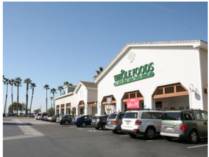
The Marina Shores shopping center has a mix of retailers serving the neighborhoods of the SEASP area.
