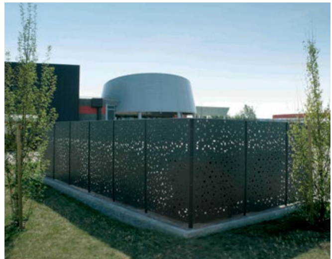
Metal screen used to screen utility area. Source: idmetalco.com
