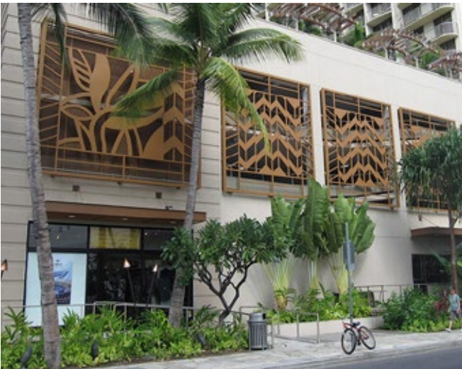
Parking structure screened with decorative panels.
